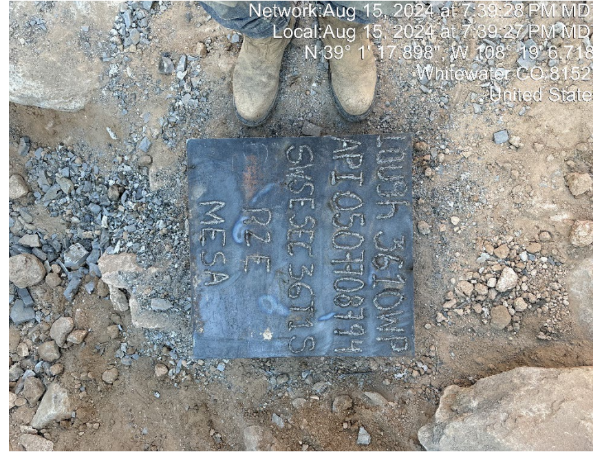
Well cut and cap plate.
