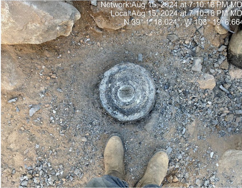
Cement to surface.
