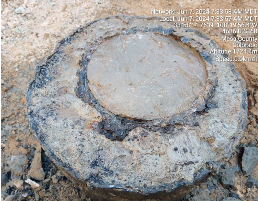
Cement to surface.
