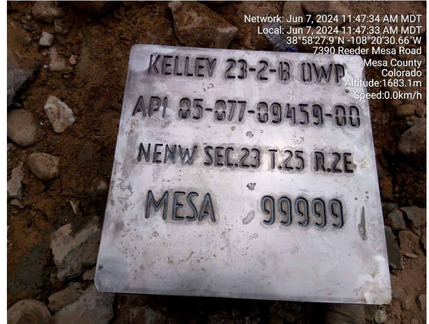
Well cut and cap plate.
