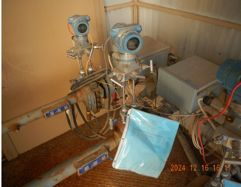
7. Gas meter inside remote meter shed.
