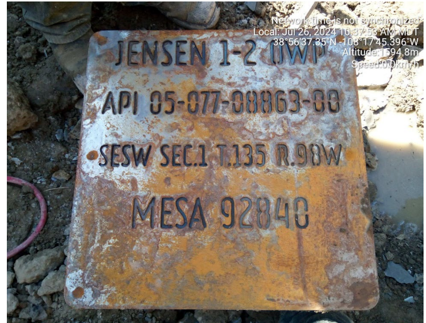
Well cut and cap plate.
