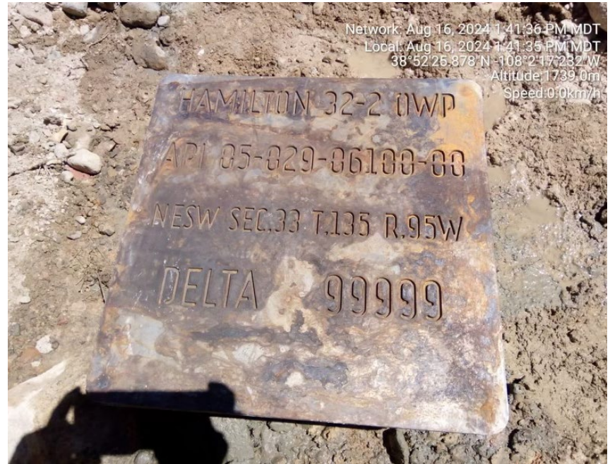
Well cut and cap plate.
