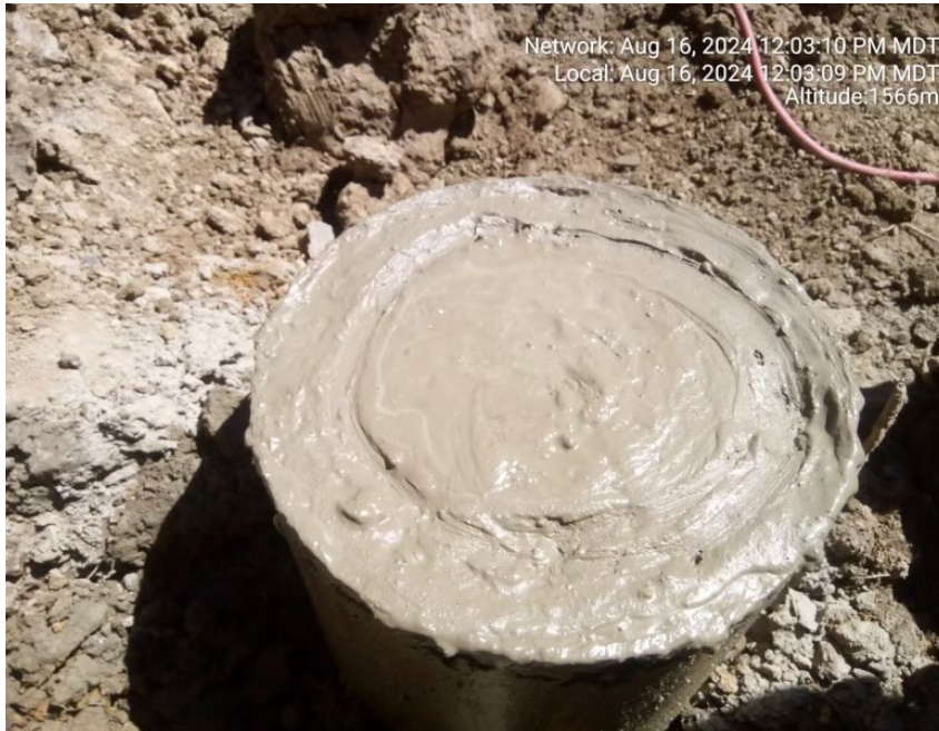
Cement to surface.
