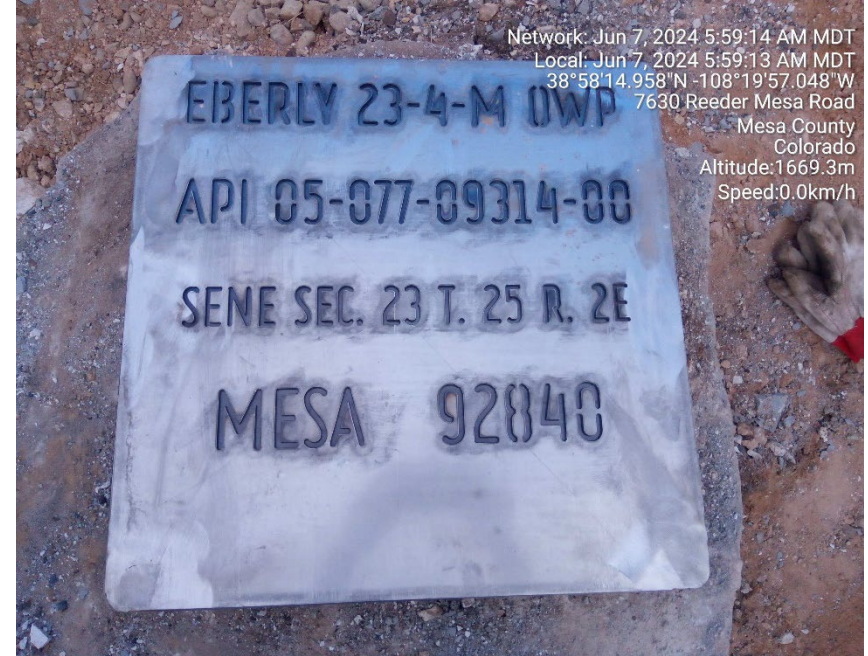
Well cut and cap plate.
