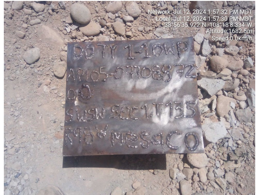
Well cut and cap plate.
