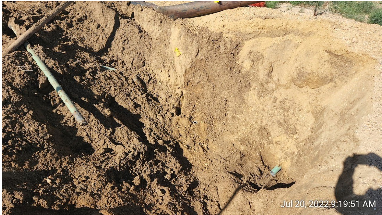
#1E – PTF C 32-8 Flowline Removal – 8FL06@4.0' – Separator Tie-in – No Impacts Noted - PID 1.0ppm
