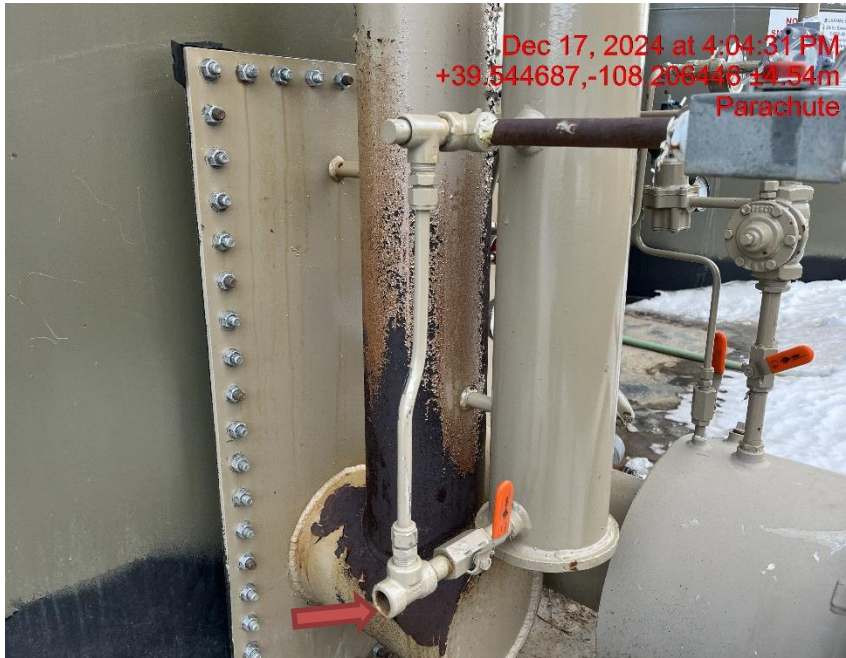
Photo # 1494 Tank heater PRV vent line does not comply with CECMC pressure safety device rules
