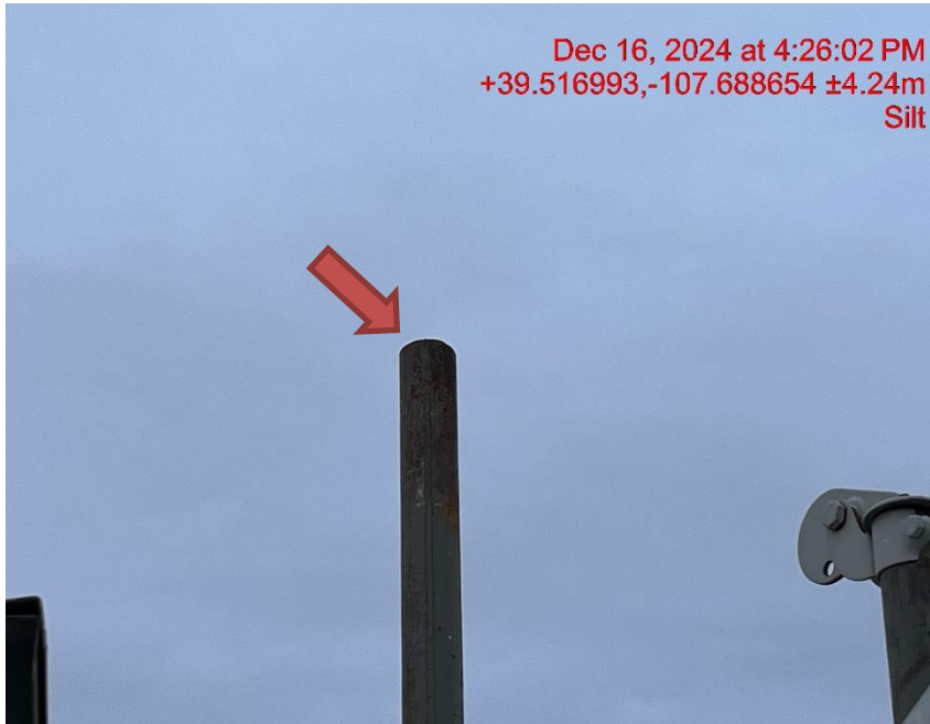
Photo # 1271 PRV vent line does not comply with CECMC pressure safety device rules
