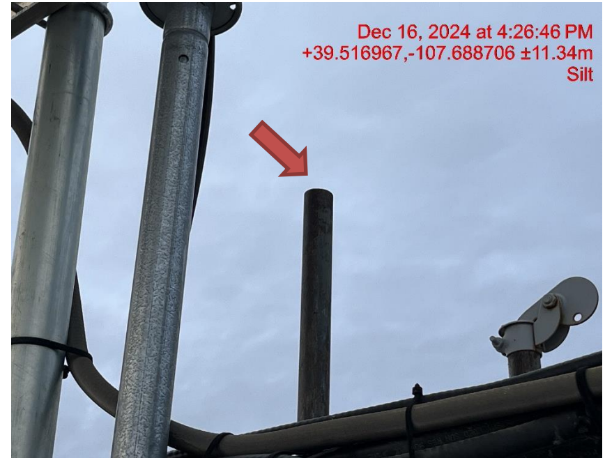
Photo # 1273 PRV vent line does not comply with CECMC pressure safety device rules
