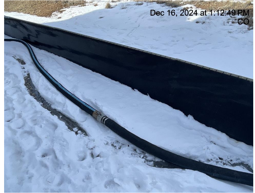
Photo # 3851 Unused hoses in secondary containment
