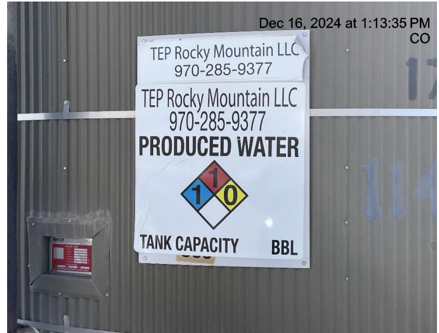
Photo # 3853 Tank label lacks capacity
