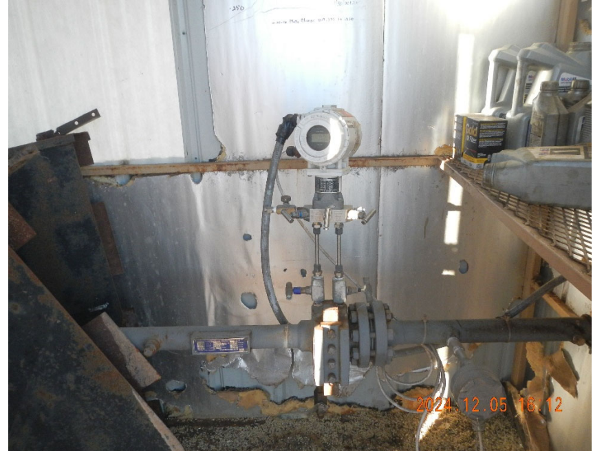
6. Gas meter inside meter shed.
