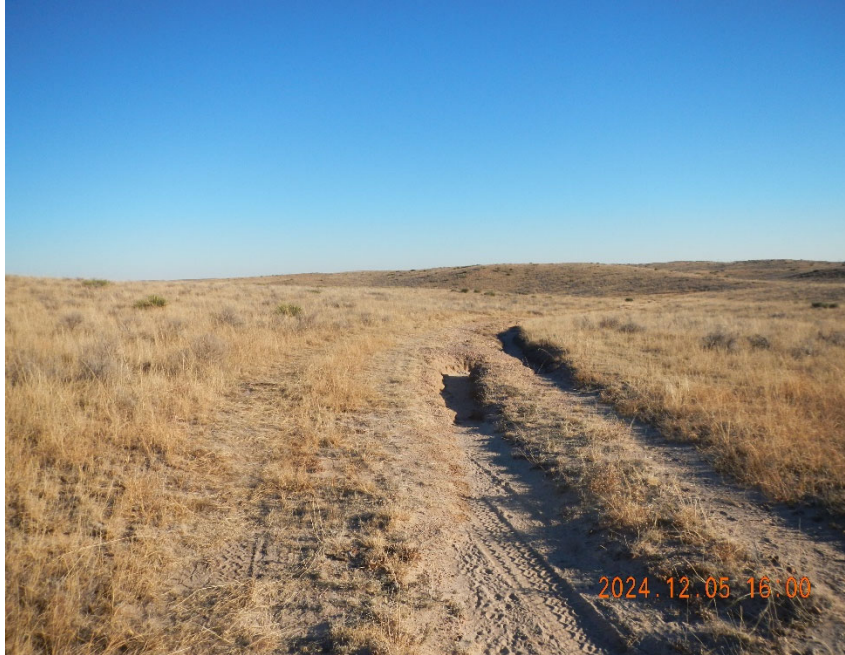
7. Erosion channeling on access trail.
