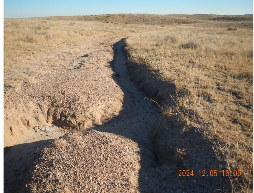
8. Erosion gulley's cut into access trail.
