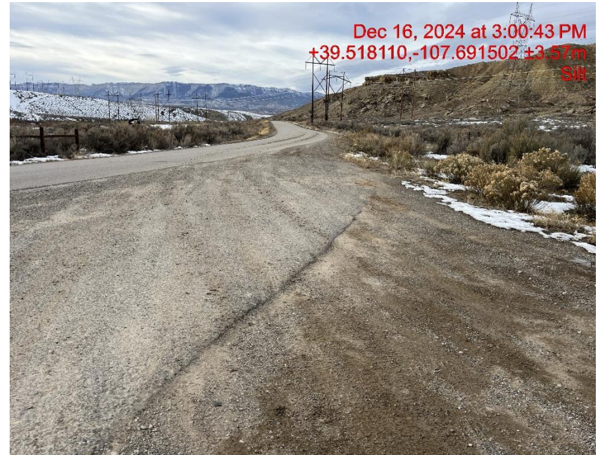
Photo # 1171 Insufficient tracking BMP's/tracking off location & onto to Mamm Creek Rd
