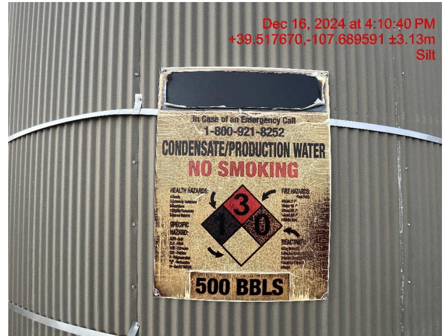
Photo # 1246 Tank label is weathered & some required information is illegible/does not comply with CECMC labeling rules
