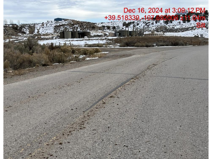
Photo # 1188 Insufficient tracking BMP's/tracking off location & onto to Mamm Creek Rd
