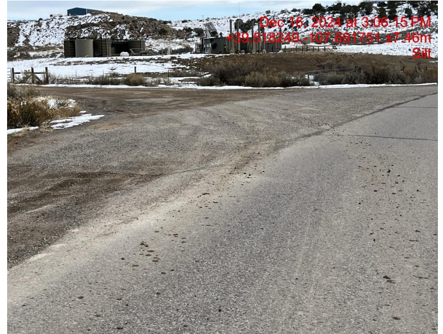
Photo # 1180 Insufficient tracking BMP's/tracking off location & onto to Mamm Creek Rd
