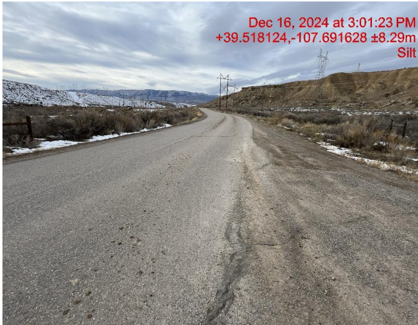
Photo # 1175 Insufficient tracking BMP's/tracking off location & onto to Mamm Creek Rd
