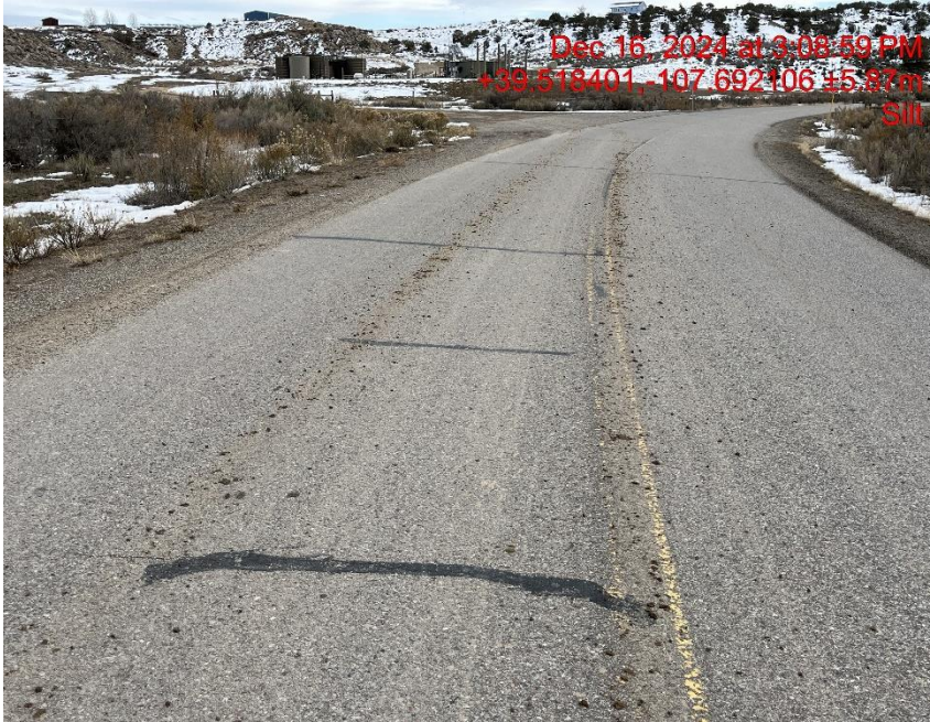
Photo # 1187 Insufficient tracking BMP's/tracking off location & onto to Mamm Creek Rd
