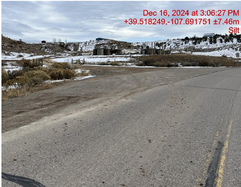
Photo # 1181 Insufficient tracking BMP's/tracking off location & onto to Mamm Creek Rd
