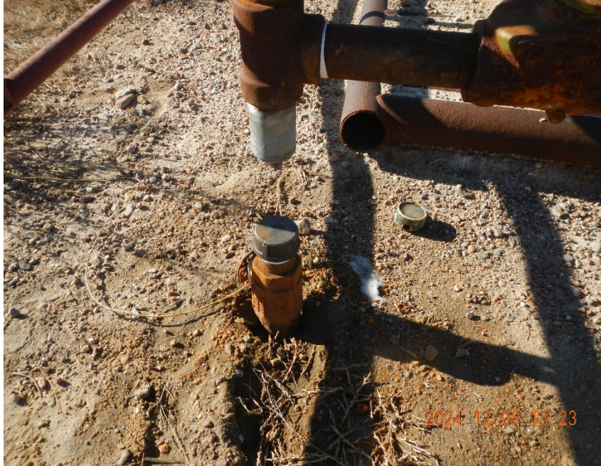
3. View of repair work completed removing broken gauge.
