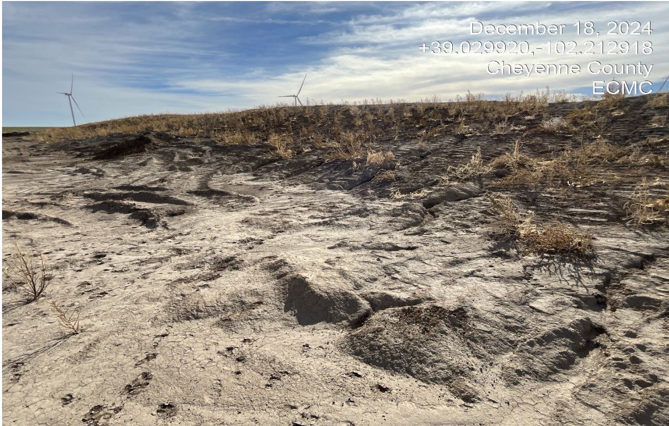
Photo 7. The topsoil pile at the west side of the location has not been protected from erosion and weeds. Topsoil needs to be replaced back for interim reclamation.
