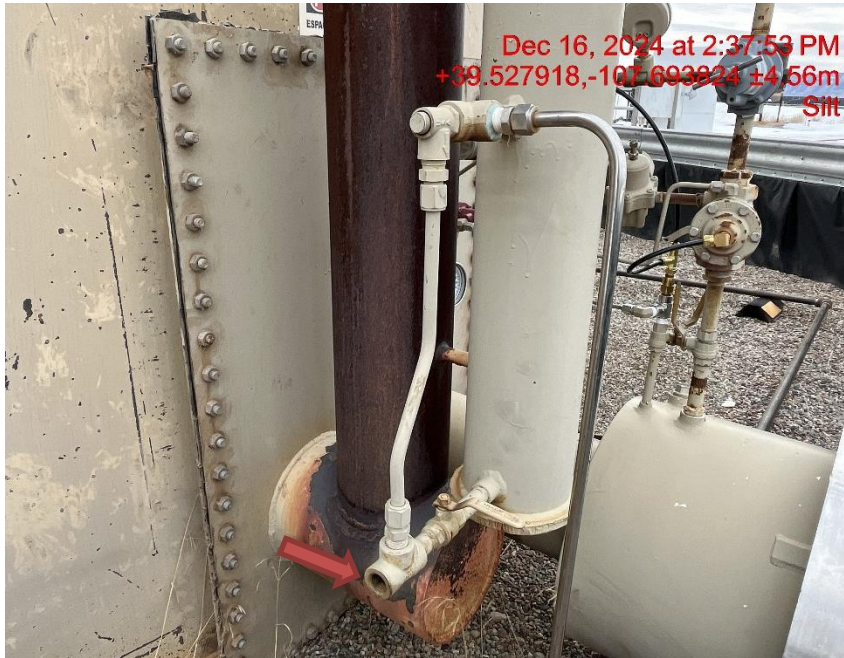
Photo # 1154 PRV vent line does not comply with CECMC pressure safety device rules
