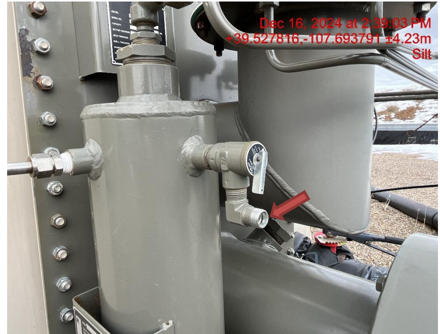
Photo # 1156 PRV vent line does not comply with CECMC pressure safety device rules
