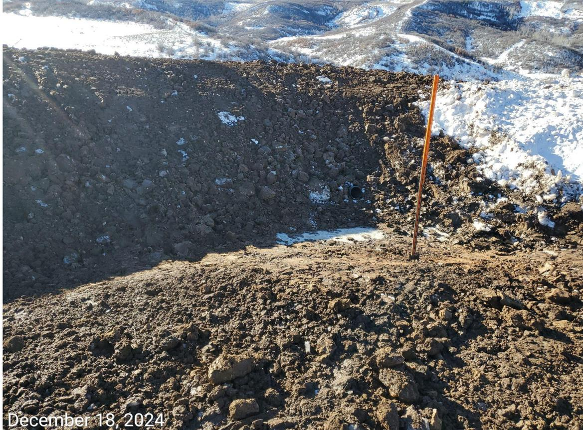
**Photo 13:** Photo shows slope drain installed on the southwest end of the pad. Slope drains on the Location have not been installed with a properly engineered and armored Inlet/outlet, including inlet/outlet protections.
