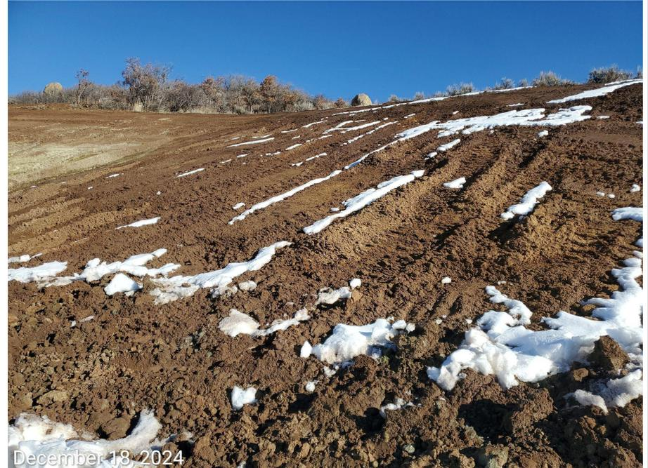
**Photo 14:** Photos taken from the cut slopes on the east/northeast end of the Location. Photos examples showing BMPs to stabilize the slopes, as well as to minimize erosion and degradation remain missing or insufficient.
