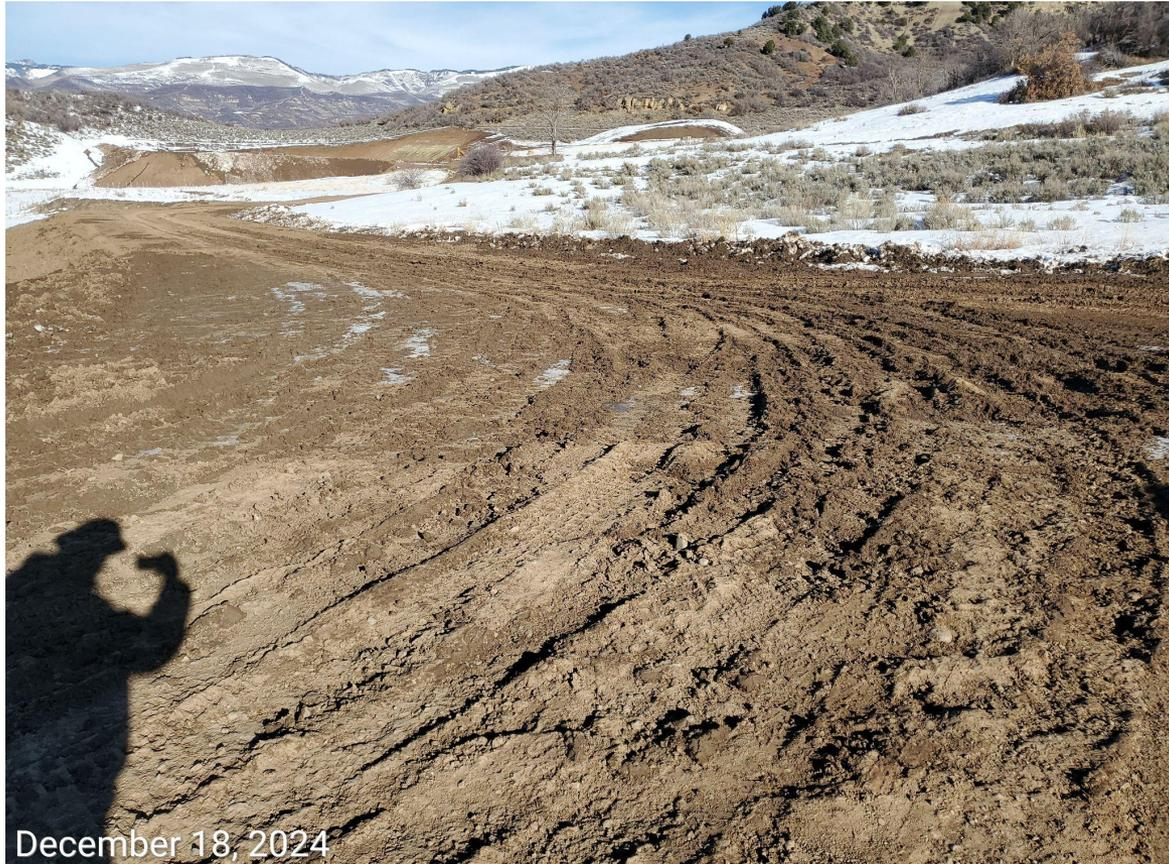
**Photo 20:** Photo taken from the access road. BMPs to stabilize, as well as to minimize tracking, degradation and sediment transport remains missing or insufficient.
