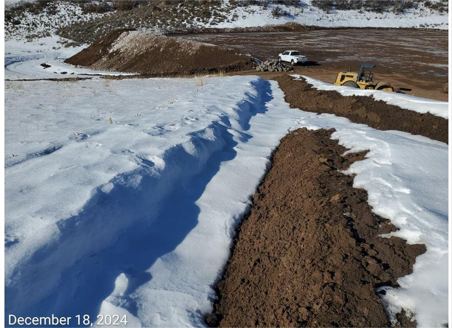
**Photo 4:** Photos taken from the southeast end of the Location. Photo shows perimeter stormwater diversion ditch has been completed. Photo right also shows culvert and sediment trap installed at ditch/location entrance; BMP has not been constructed with properly engineered inlet/outlet protections.
