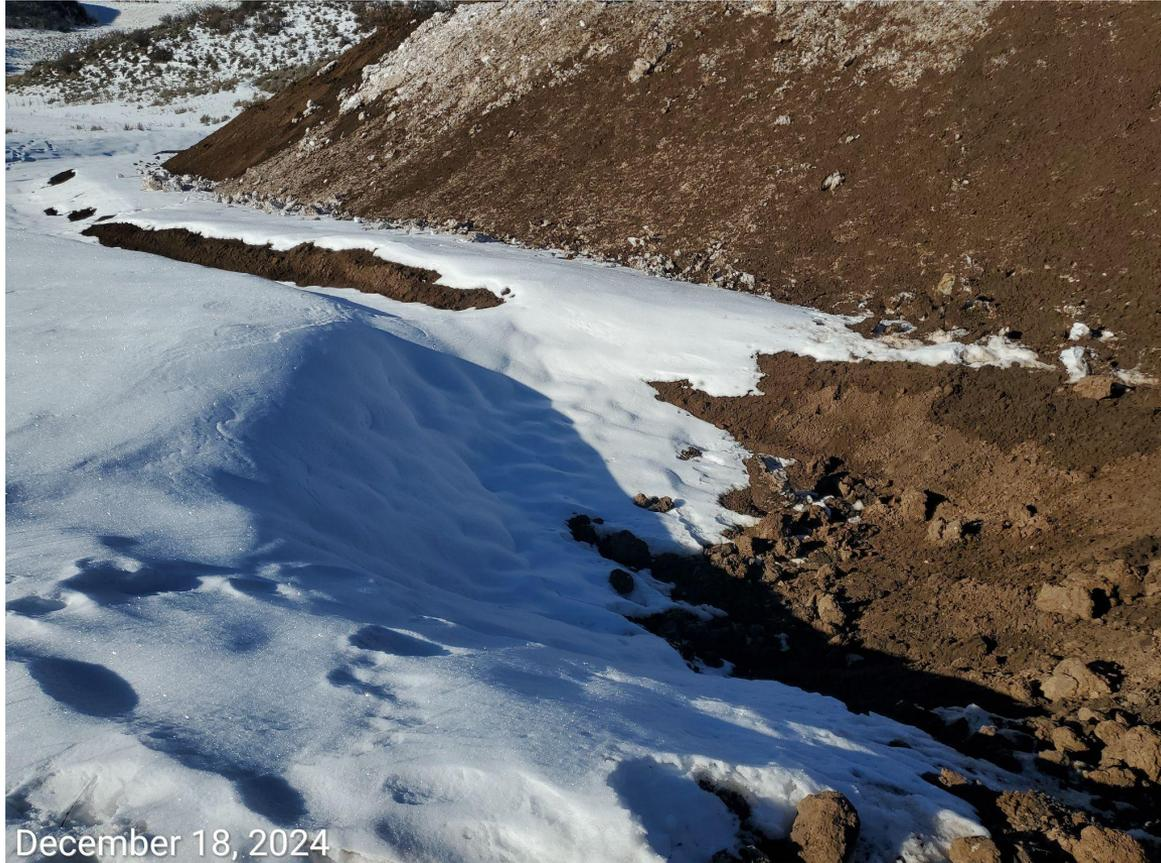
**Photo 6:** Continued from photo 5. Sediment trap at culvert has not be installed/constructed with properly engineered inlet/outlet protections.
