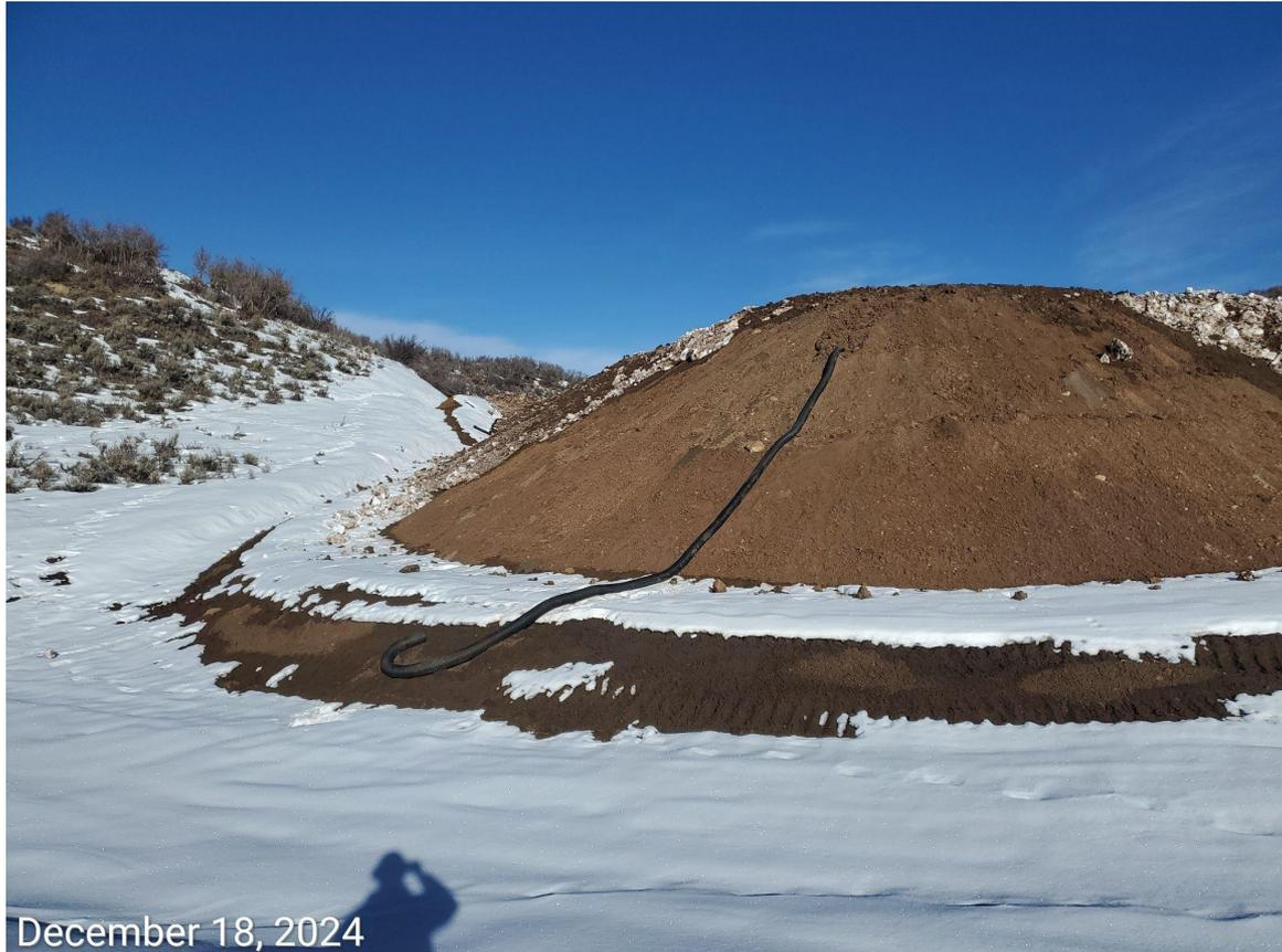
**Photo 8:** Photo taken from the southwest end of the Location. Operator has installed a slope drain; BMP has not been secured, or constructed with a properly engineered and armored outlet.
