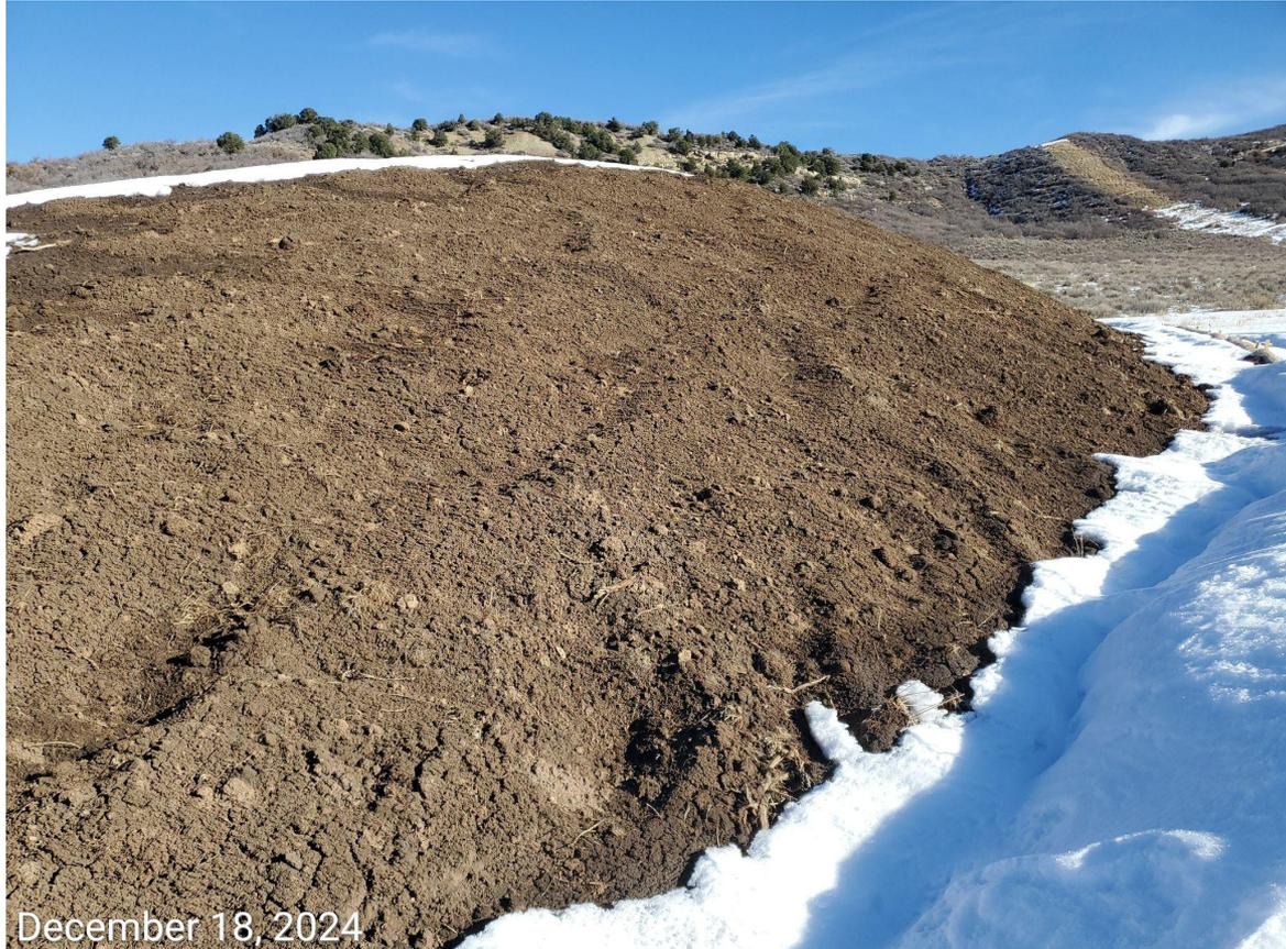
**Photo 15:** Photo taken from the topsoil stockpile on the east end of the Location. Photos examples showing BMPs to stabilize the slopes, as well as to minimize erosion and degradation remain missing or insufficient.
