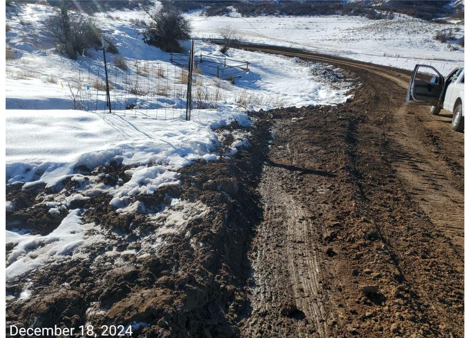
**Photo 18:** Photos taken from along the access road. Photo shows that the 24" Culvert in conjunction with "Trap w/ rock armored rundown" has not been installed along the access road between the stockpond and the Location entrance pursuant to the Form 2A permitted SWMP and Layout Drawing.
