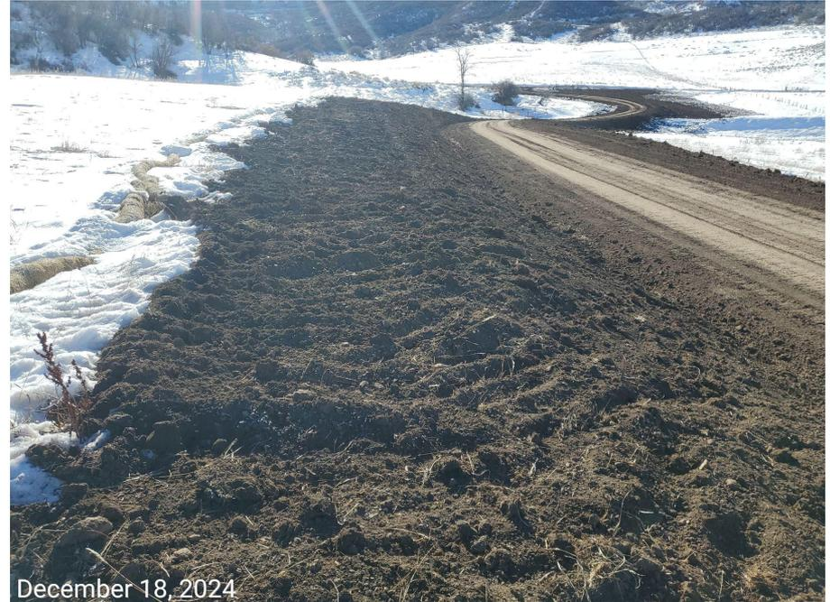
**Photo 16:** Photos taken from the access road. Road has been contoured and erosion logs have installed upslope. Photos also show that the topsoil remains bare and exposed; BMPs to stabilize the slopes, as well as to minimize erosion and degradation remain missing or insufficient.
