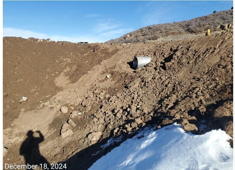
**Photo 5:** Photos taken from the Location entrance on the south end of the Location. Photos show culvert and sediment trap(s) have been installed at the location entrance; BMP has not been constructed with properly engineered inlet/outlet protections.
