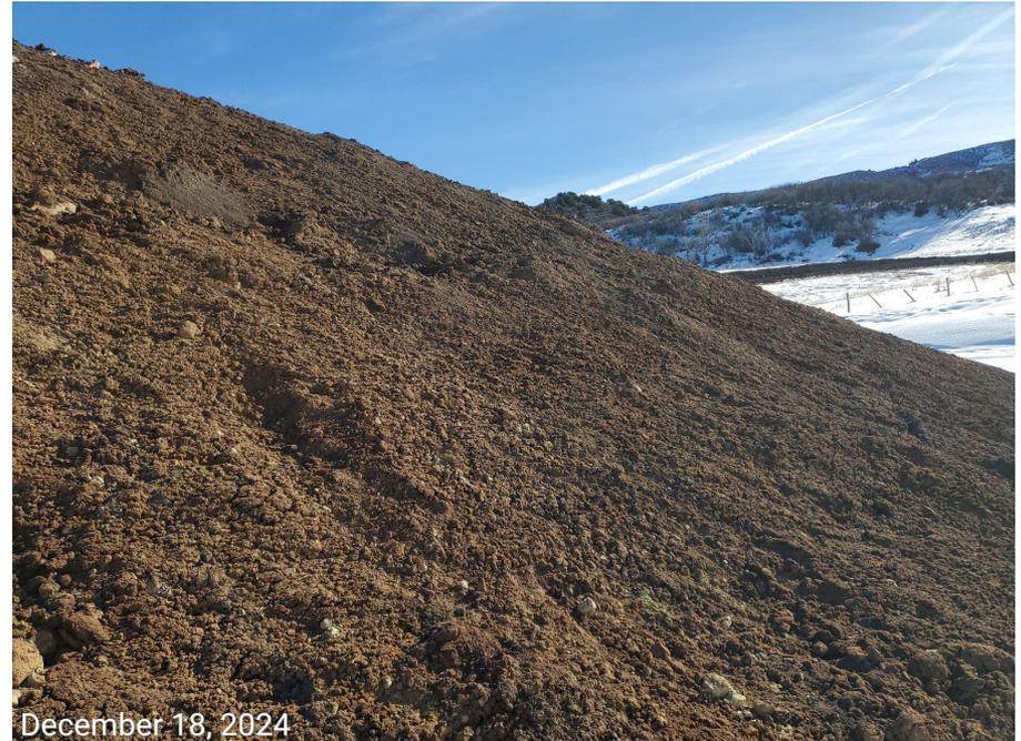
**Photo 9:** Photos taken from the fill slopes on the southwest end of the Location. Photos examples showing BMPs to stabilize the slopes, as well as to minimize erosion and degradation remain missing or insufficient.
