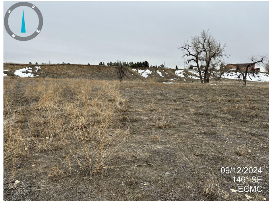
Photo 2. Photo taken looking southeast across wellsite. Undesirable weedy vegetation is present and poor vegetation coverage.
