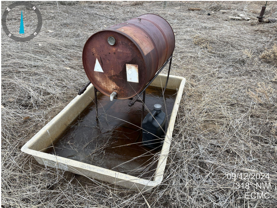
Photo 11. No wildlife exclusion device on secondary containment.
