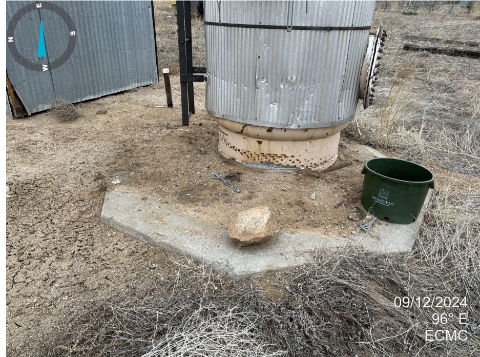
Photo 4. Stained soil remains at separator.
