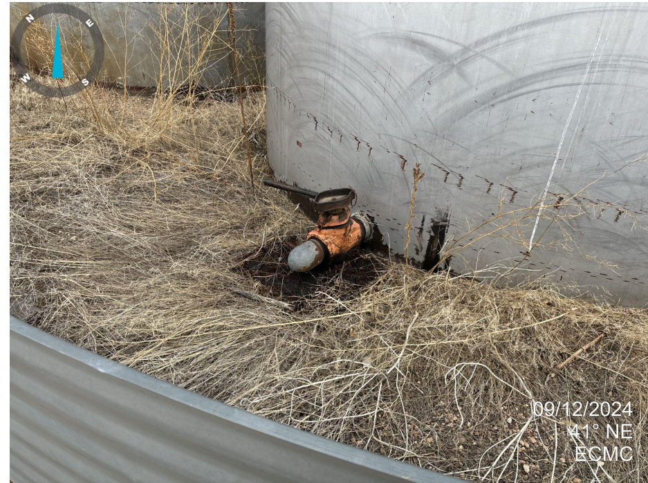
Photo 2. Stained soil and oily waste at southern tank valve. Weeds present within secondary containment.
