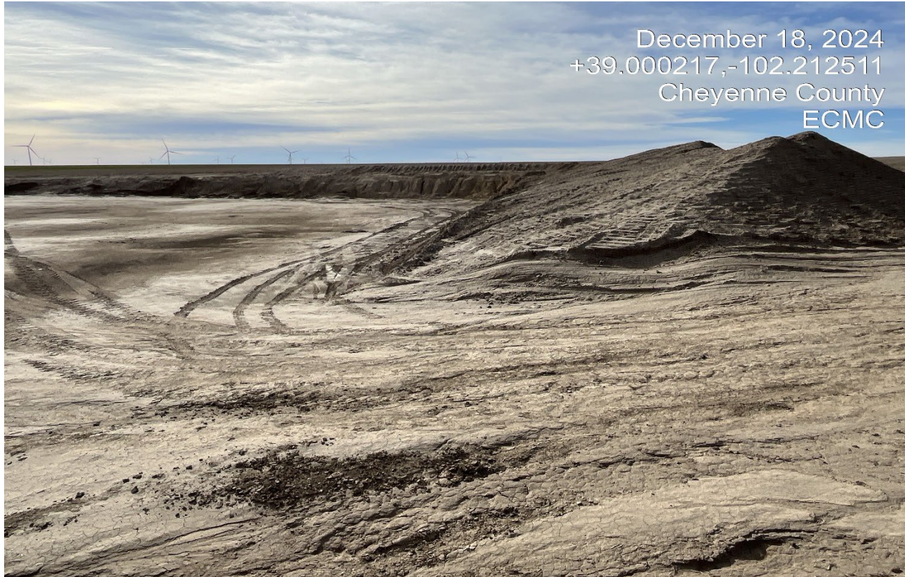
Photo 3. North side of the location facing east. Topsoil is stored along the north side of the location and has not been stabilized or replaced for interim reclamation.
