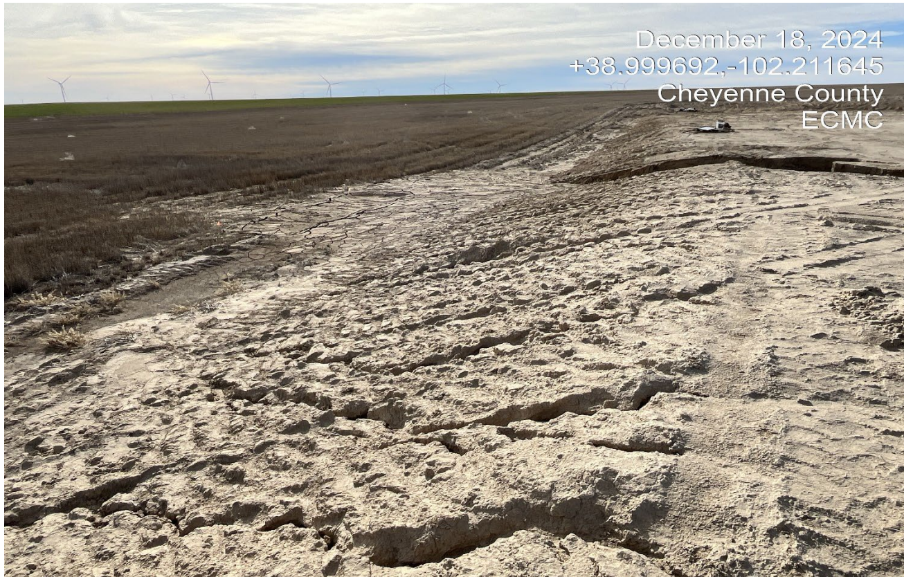
Photo 7. Facing southwest toward the fill slope which has eroded and transported sediment offsite.
