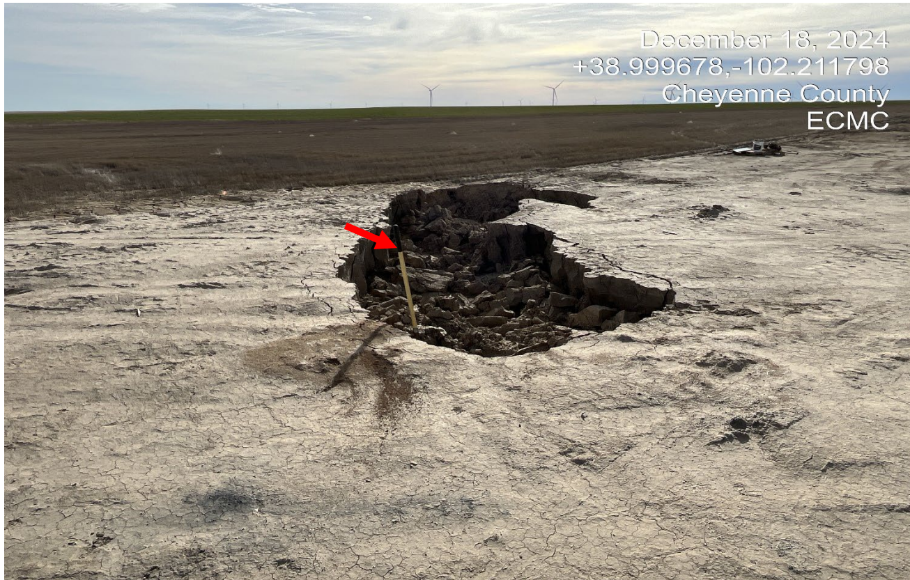
Photo 6. There is signiant gully erosion along the fill slope which has washed sediment out into the adjacent crop field. Red arrow points to 4.5 ft. shovel.
