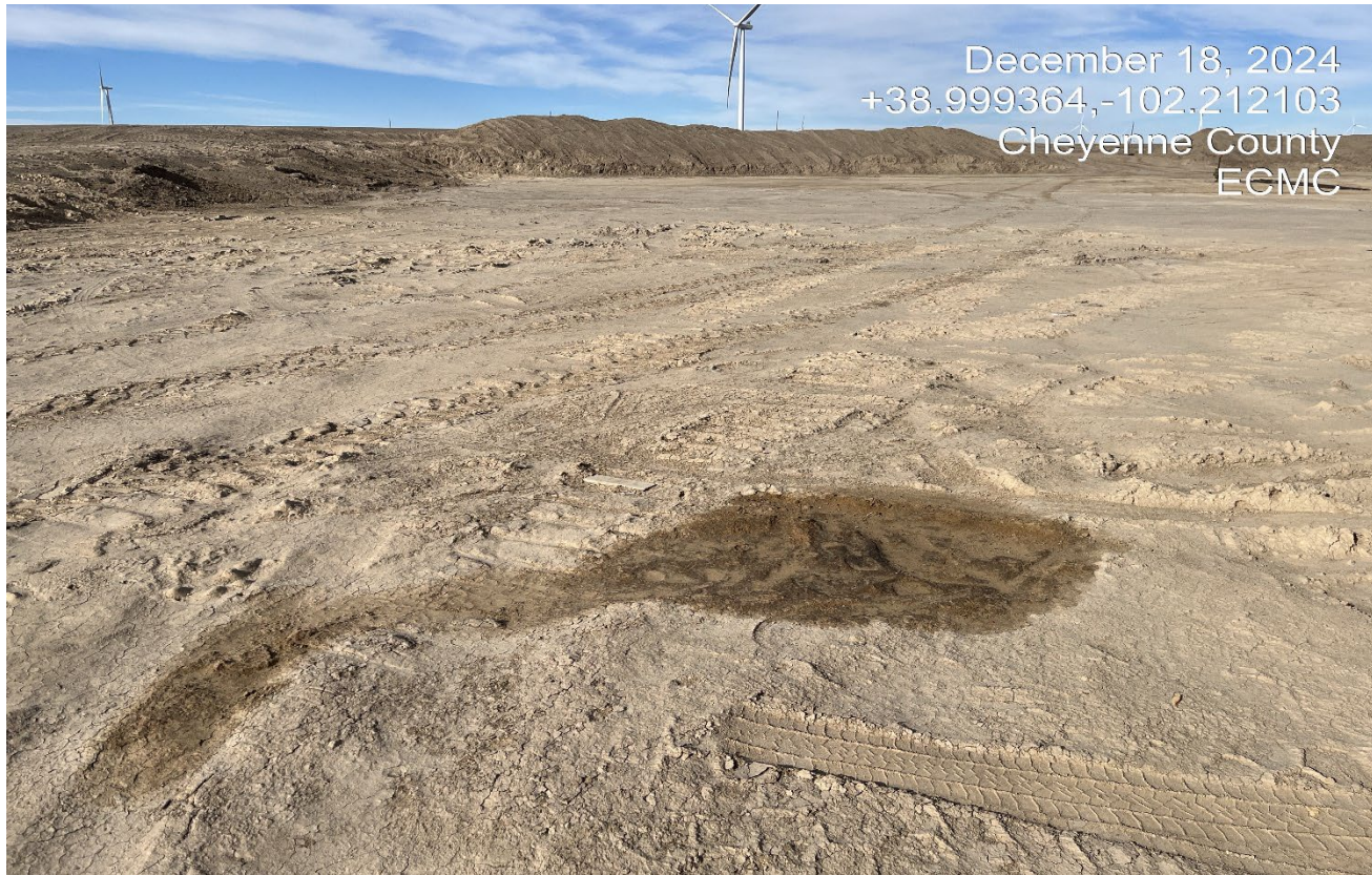
Photo 10. There is a spill and stained soils at the southwest corner that must be cleaned up.
