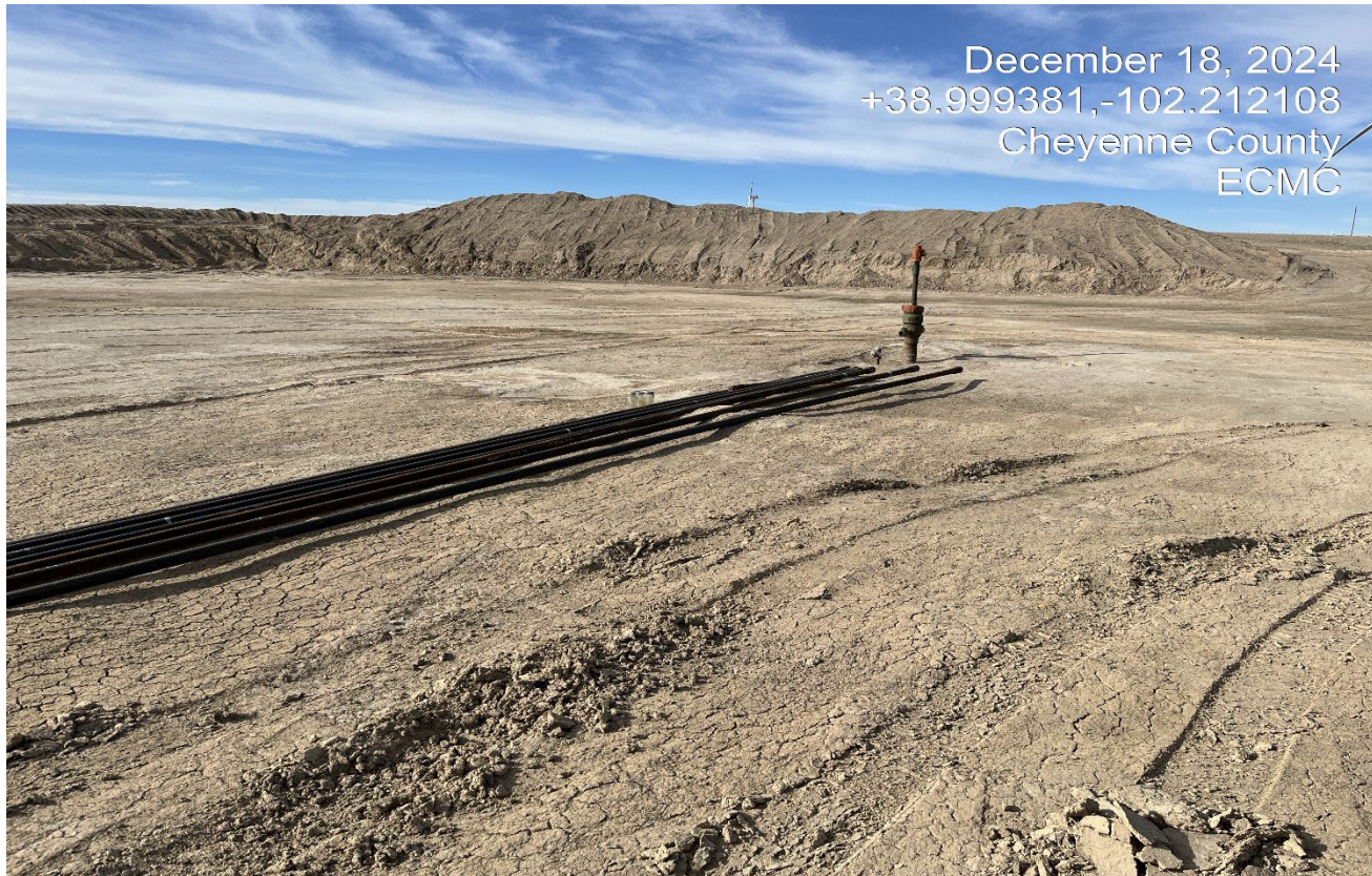
Photo 5. There is unused pipe at the wellhead that needs to be removed. There is no sign posted at the wellhead.
