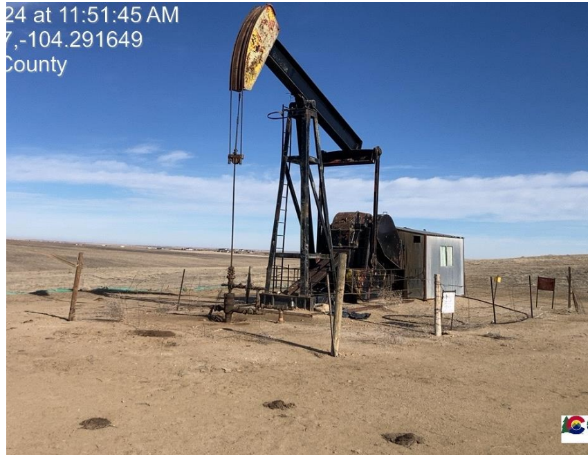
Pic 1 wellhead / pumpjack
