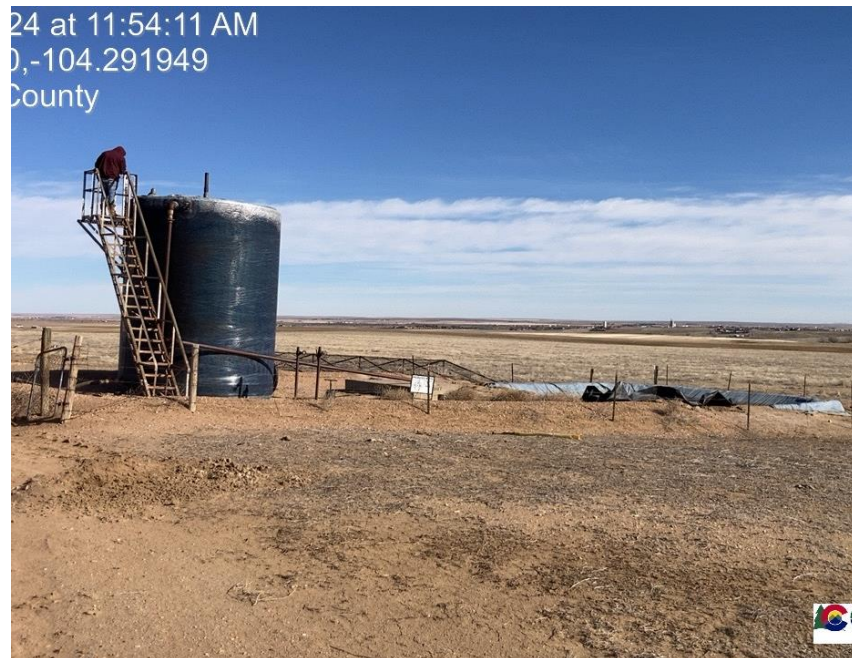
Pic 7 Water tank, pit
