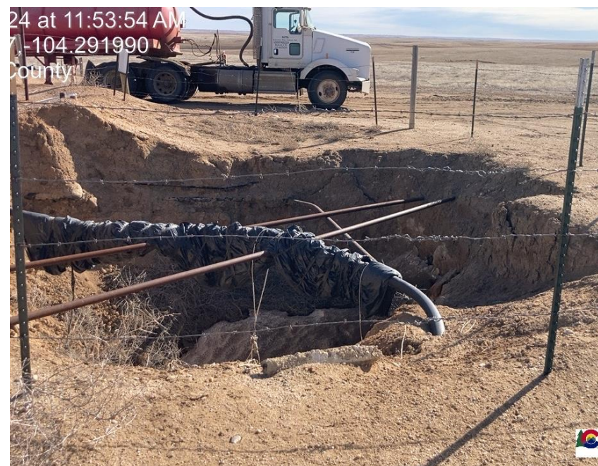
Pic 6 Open excavation
