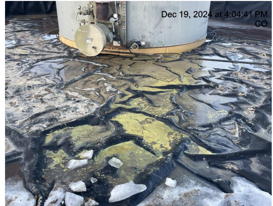
Photo # 4819 E & P/Oily waste in secondary containment
