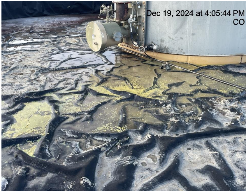
Photo # 4820 E & P/Oily waste in secondary containment
