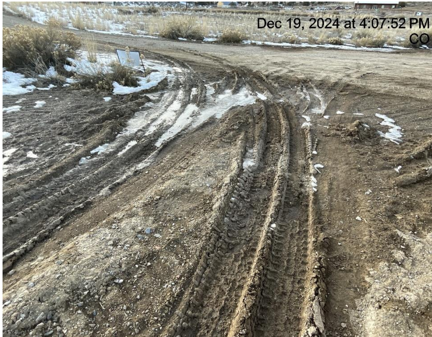
Photo # 4822 Lack of stabilization/compaction near tank battery
