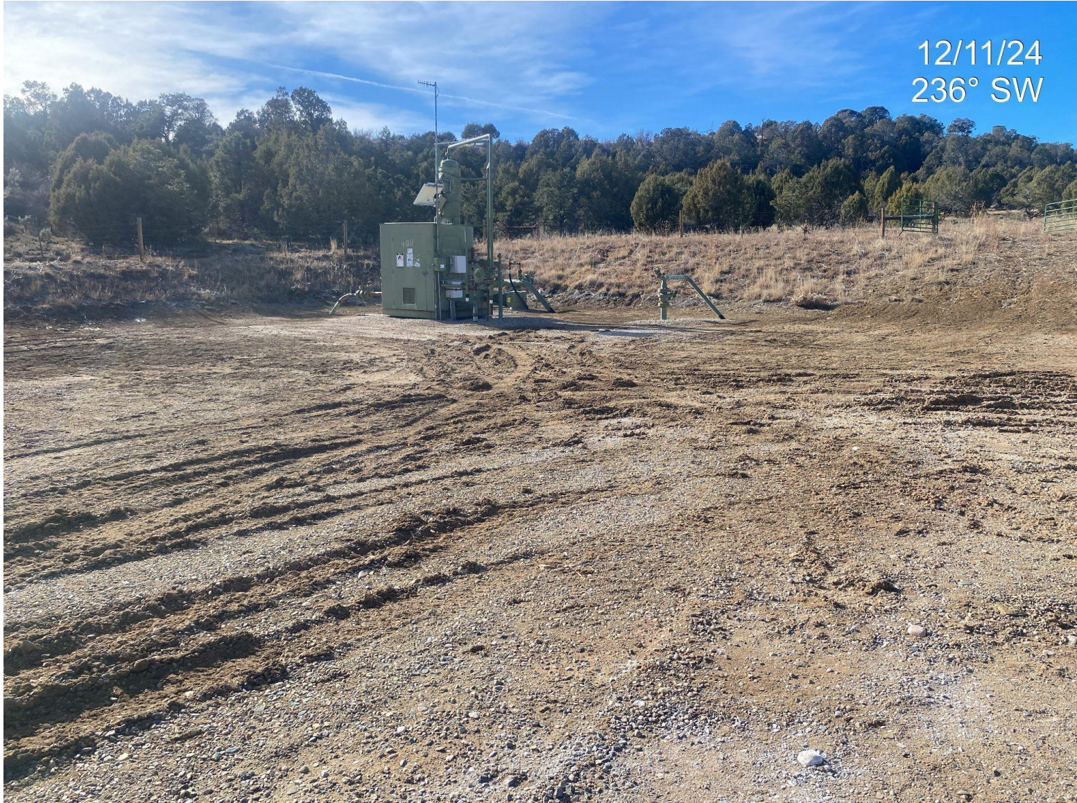
Photo 4. Rutting starting to form on pad, future maintenance is advised.
