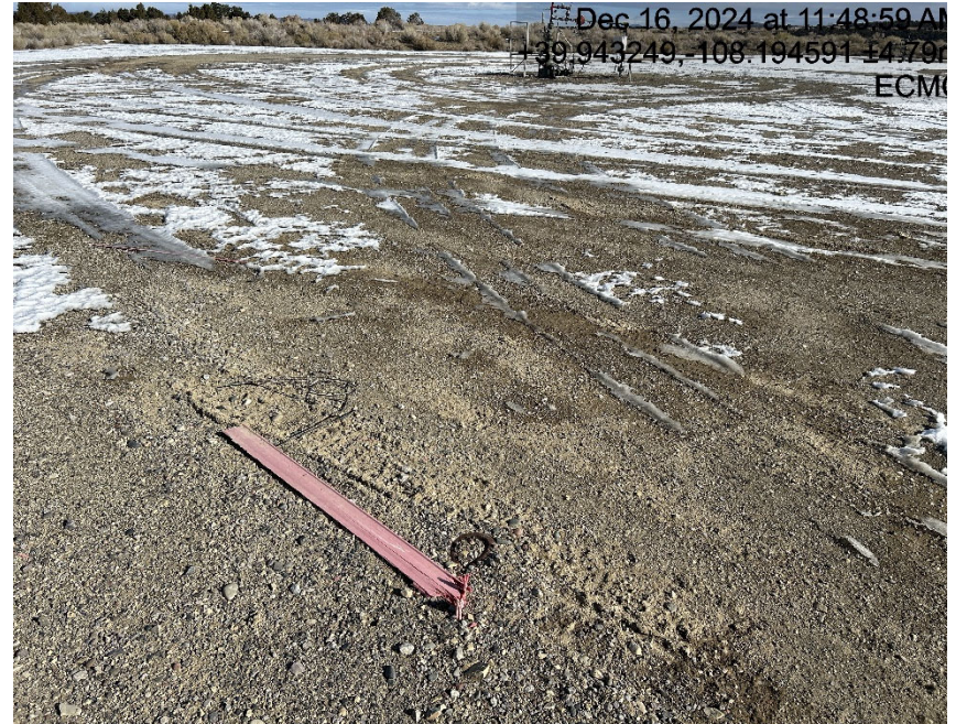
Dead man not marked properly
