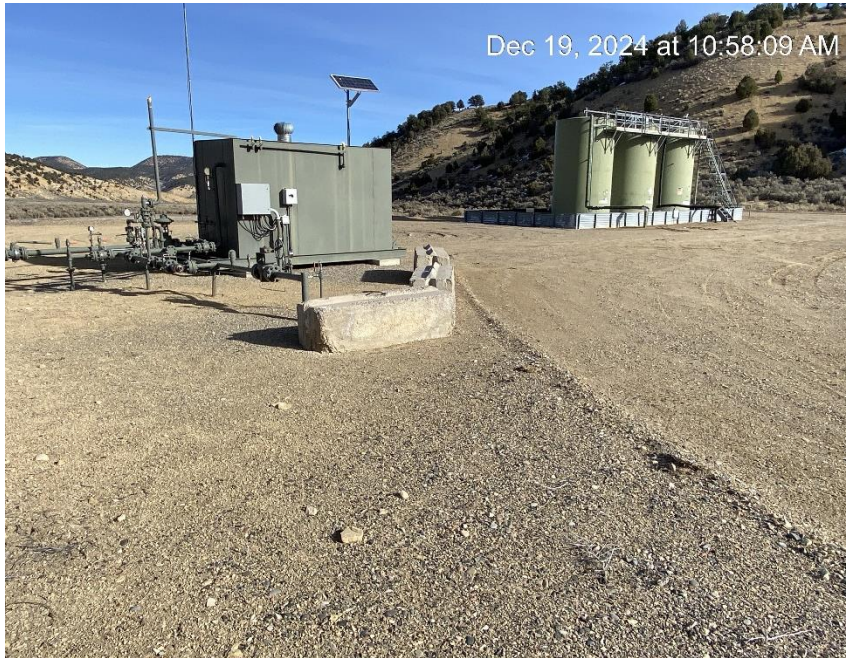
Production pad from Southwest corner
