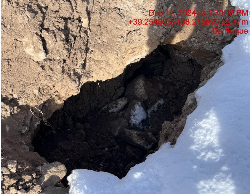
Photo # 0924 Tunnel erosion NW side of lease road near location in ditch/ditch needs maintenance, also is a wildlife/personnel safety hazard
