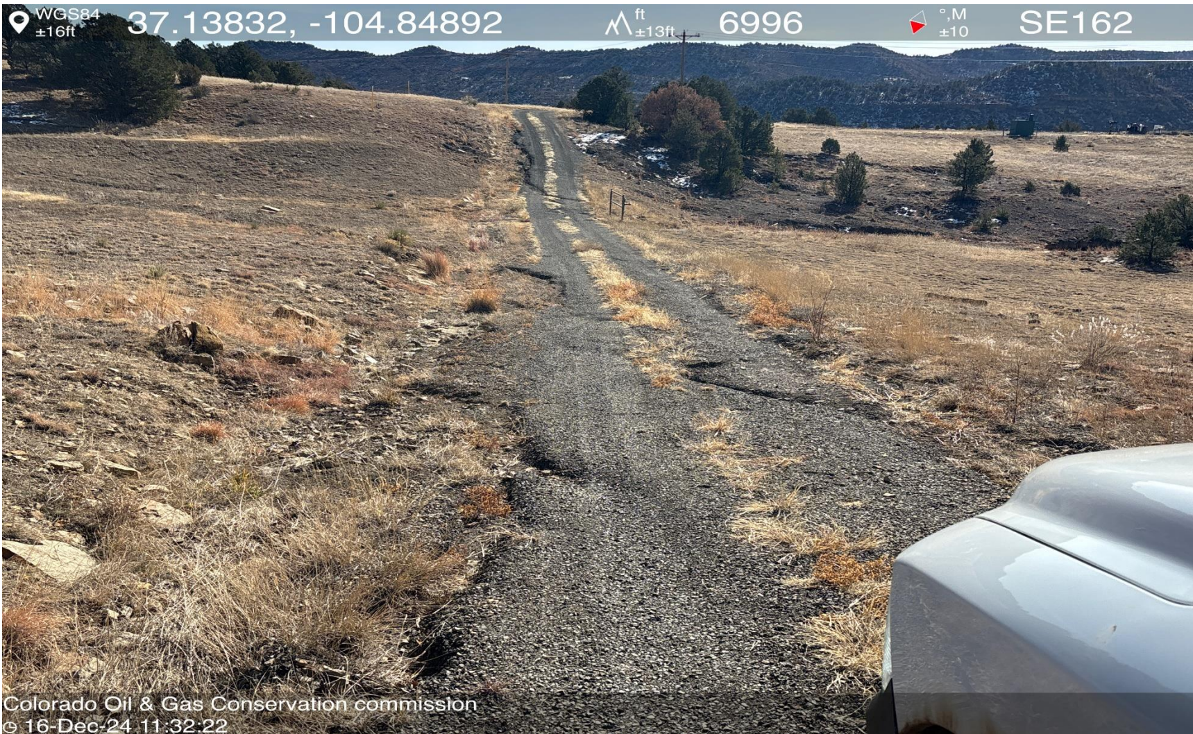
PHOTO 6: STORMWATER HAS ERODED OUT OF BMP DITCH AND HAS CAUSED CHENNELING DOWN AND ACROSS ROW IS MULTIPLE AREAS. Install or repair required BMPs per Rule 1002.f.(2)C . CA DATE 12/26/2024.
