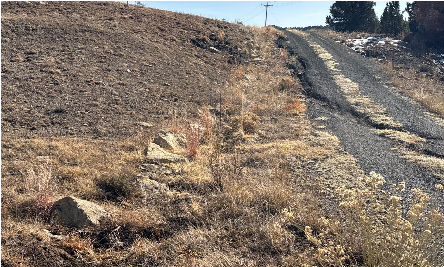
PHOTO 4: STORMWATER HAS ERODED OUT OF BMP DITCH AND HAS CAUSED CHENNELING DOWN AND ACROSS ROW IS MULTIPLE AREAS. Install or repair required BMPs per Rule 1002.f.(2)C . CA DATE 12/26/2024.
