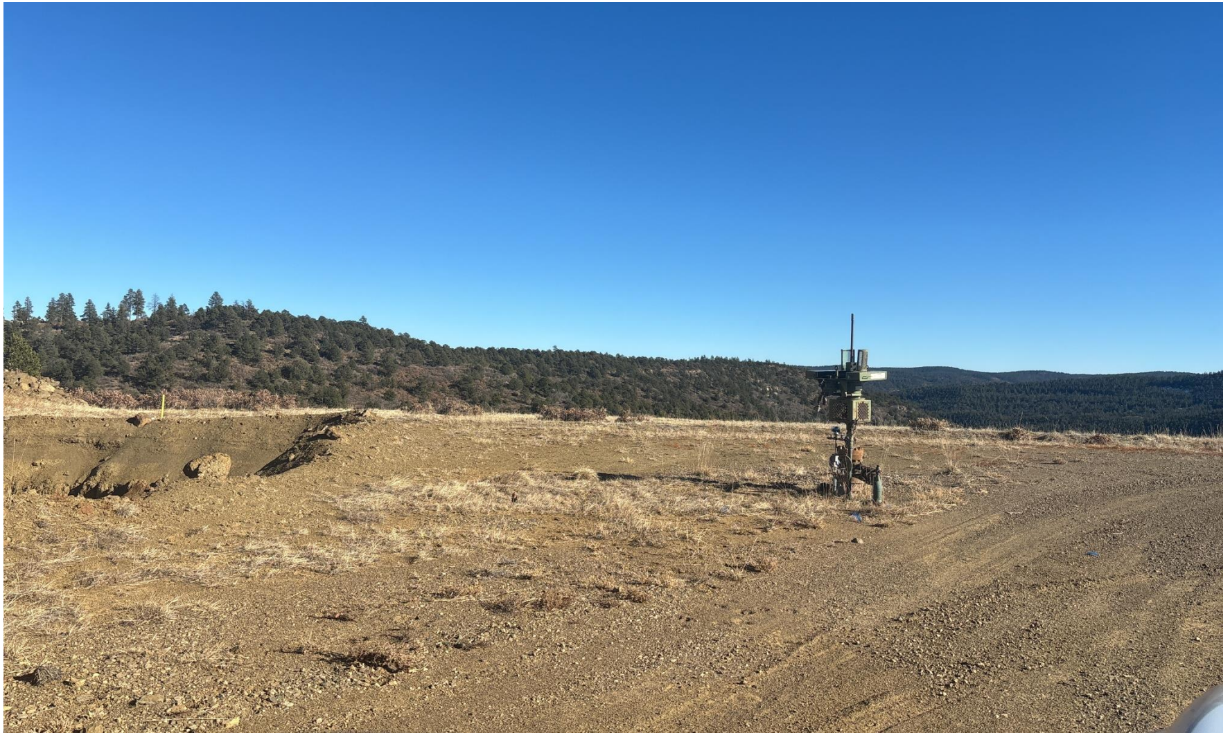
PHOTO 3: WELLHEAD AND EQUIPMENT.
