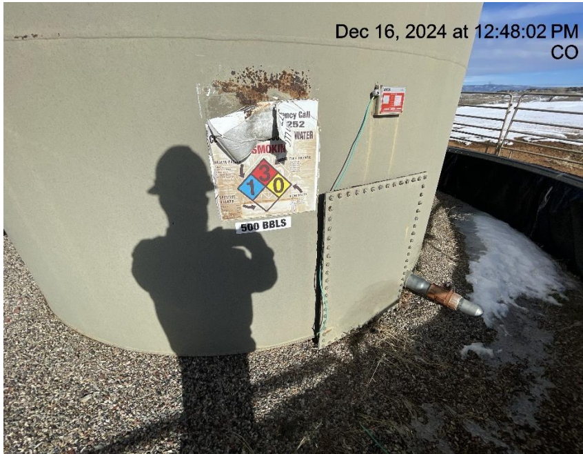
Photo # 3755 Tank label damaged & some required info is illegible
