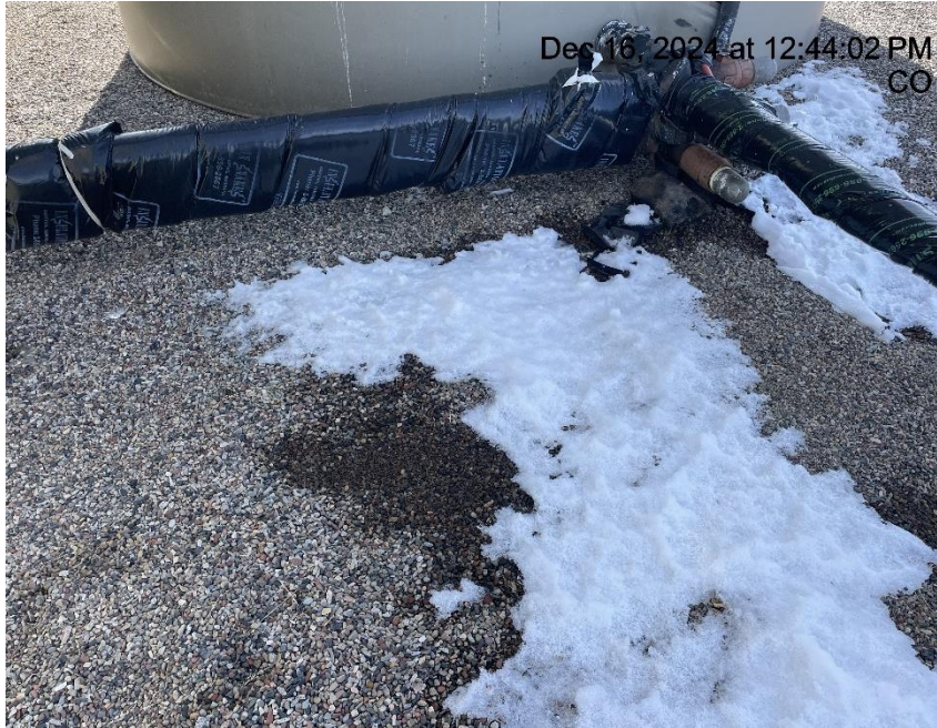
Photo # 3749 Staining in secondary containment
