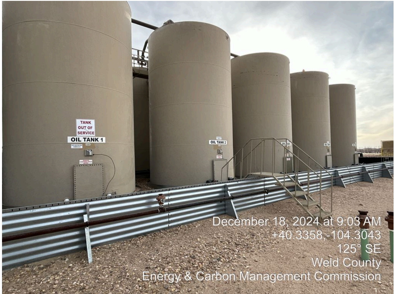
Missing Capacity Labels
