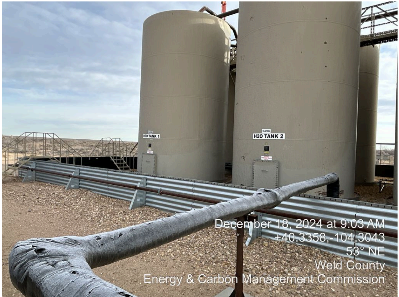
Missing Capacity Labels
