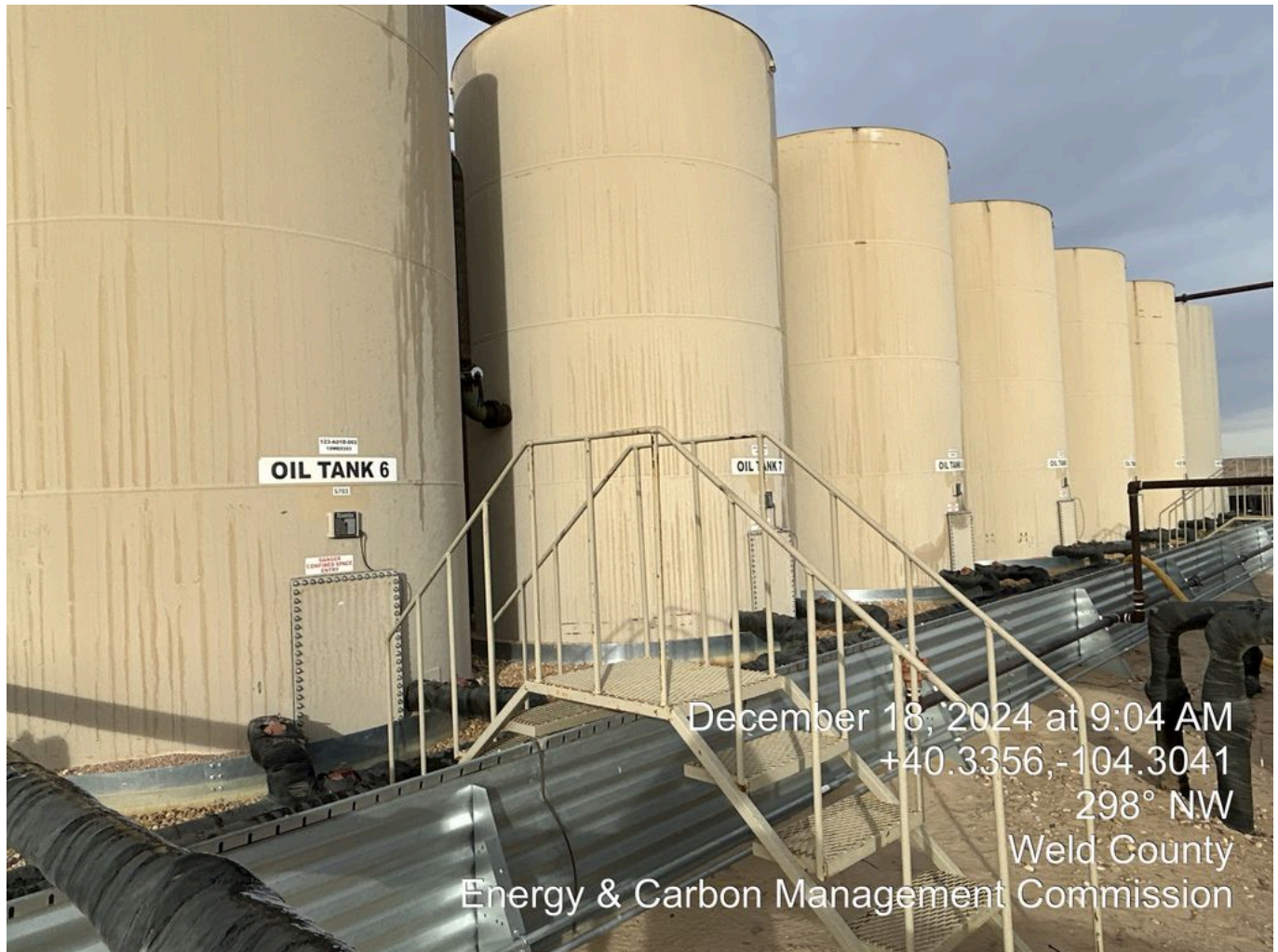
Missing Capacity Labels
