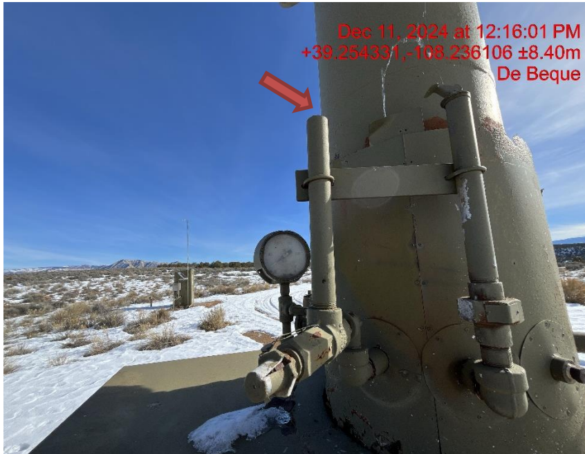
Photo # 0837 PRV vent line does not comply with CECMC pressure safety device rules
