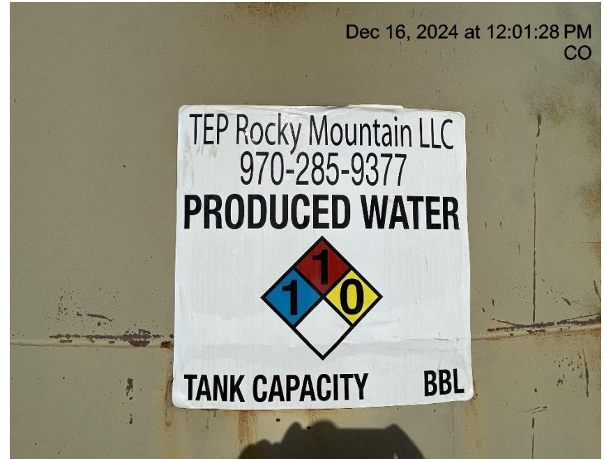
Photo # 3678 Tank label lacks capacity
