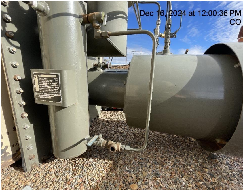
Photo # 3677 PRV vent line on tank burner does not comply with CECMC pressure safety device rules
