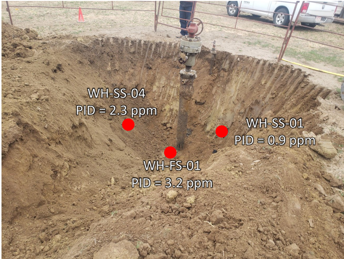
Looking northwest No petroleum hydrocarbon staining or odor observed
