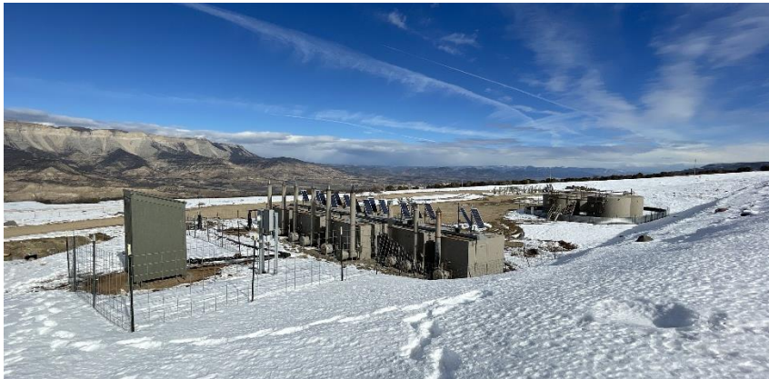
South West corner of location.
