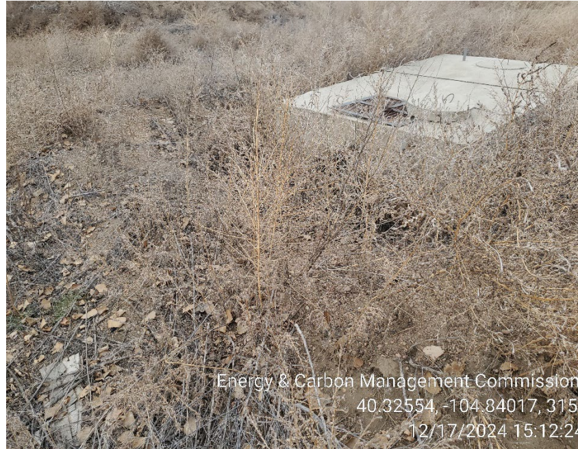
Debris and earth berm
