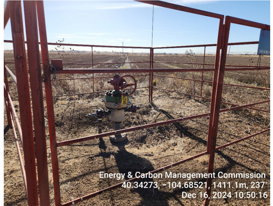
Photo 4: TA wellhead
