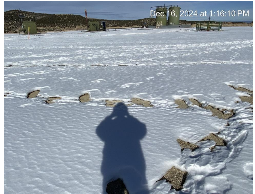
Location from South corner
