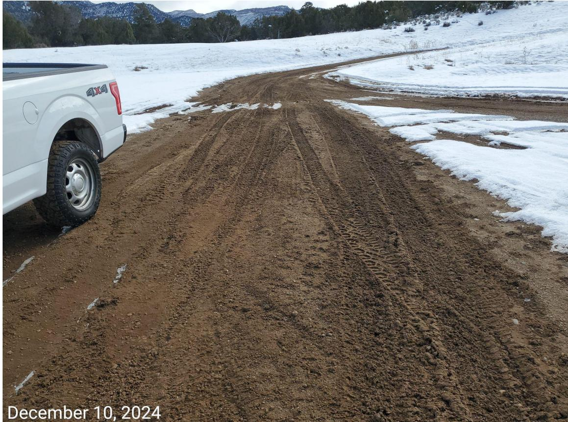
**Photo 4:** Tracking and stabilization BMP at the working pad surface show signs of disrepair. Maintenance advised to ensure control measures remain in proper functioning condition.
