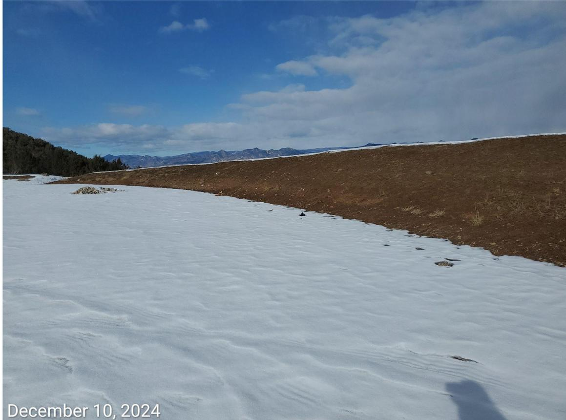
**Photo 2:** Limited inspection due to snow cover. Photo shows interim slopes of the Location that were observable during the inspection. Unable to find evidence that additional reclamation work has been performed, and BMPs to stabilize the seeded soils implemented.
