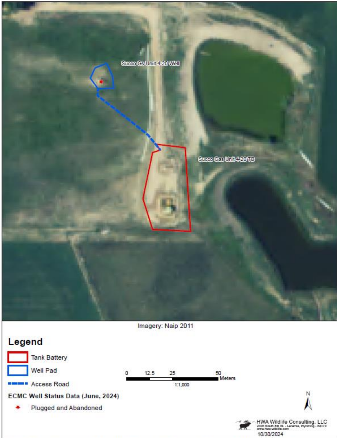
Figure 2. Pre-plugging overview of the reclaimed well site and the associated access road, tank battery, and flowline.
