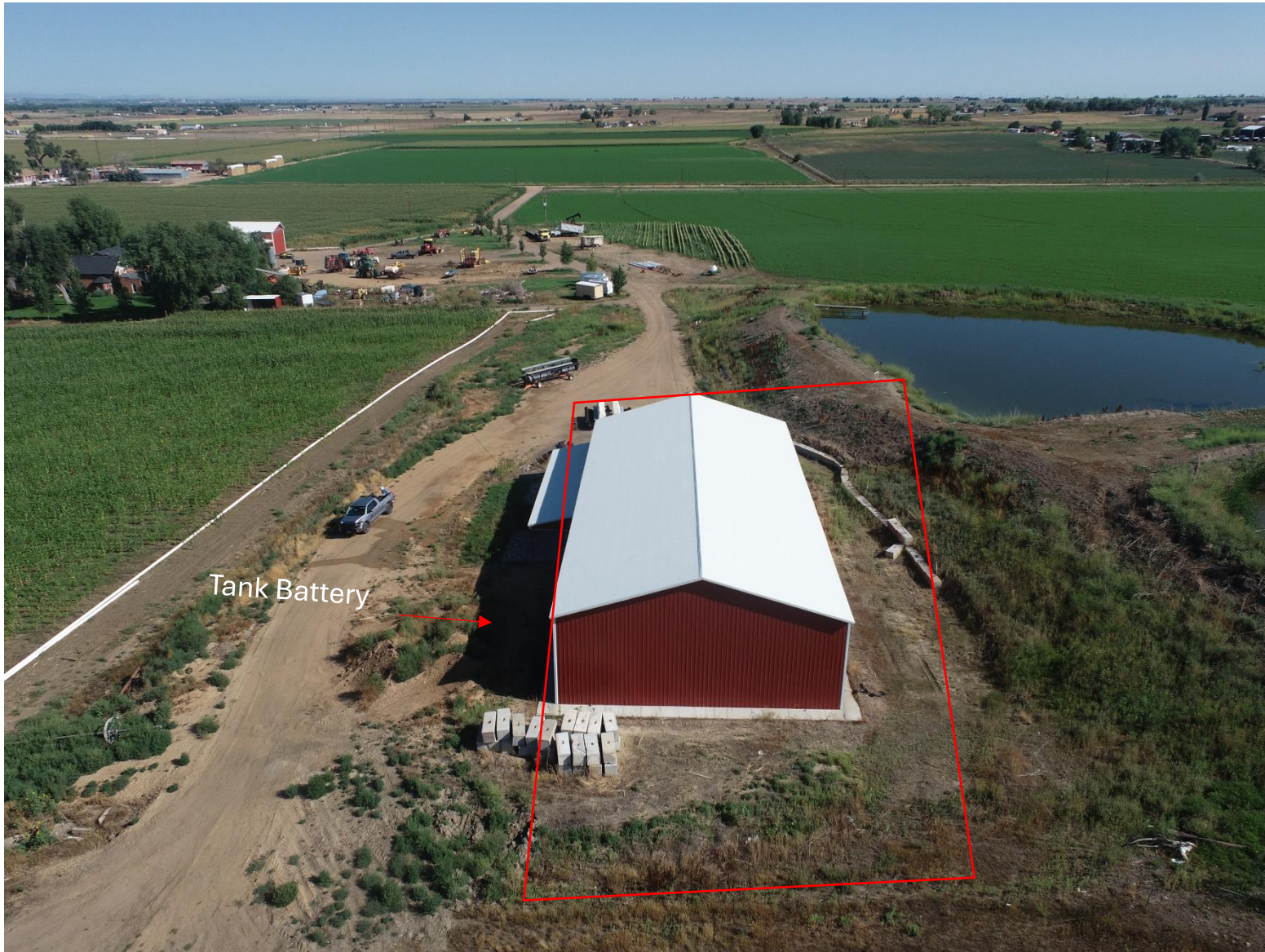
Figure 8: Looking North towards TB, 100 feet in height, Lat/Long: 40.119707/-104.79737.
