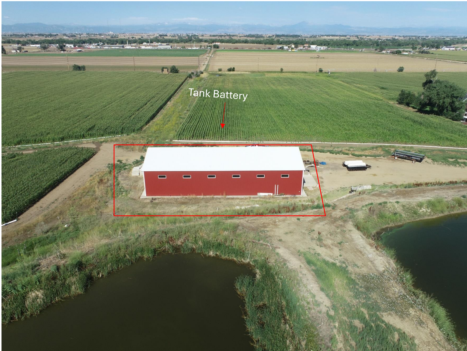
Figure 10: Looking West towards TB, 100 feet in height, Lat/Long: 40.120242/-104.796435.
