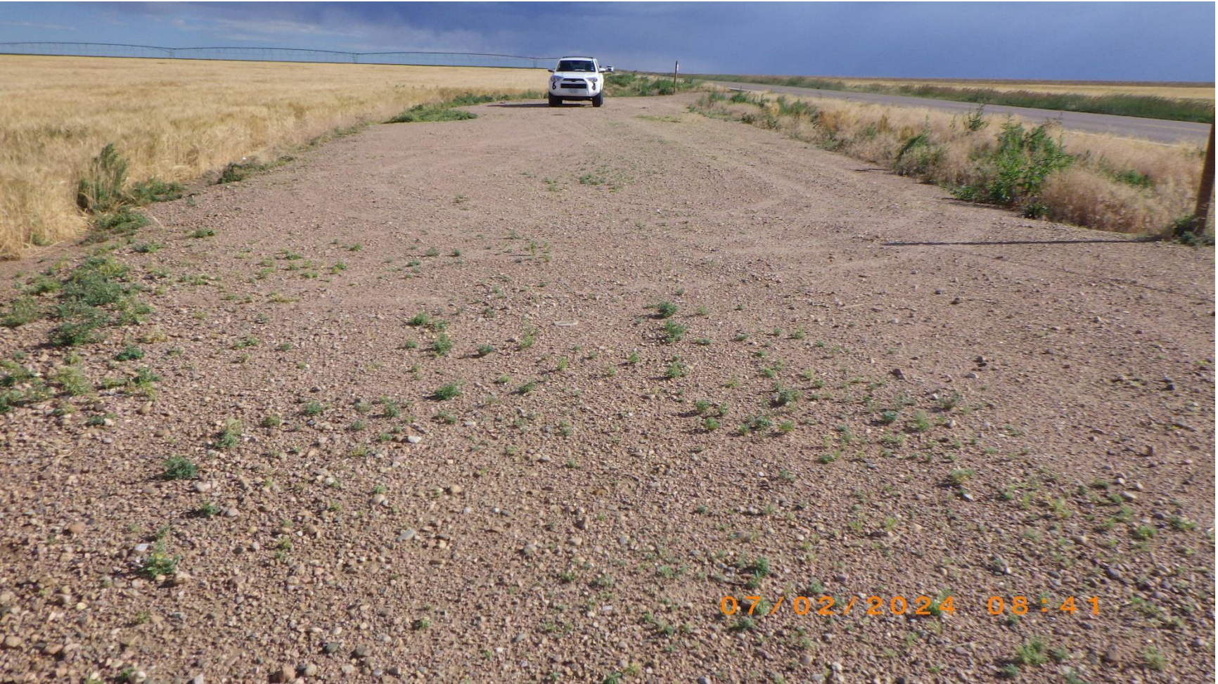
Figure 14: South edge of TB looking North.
