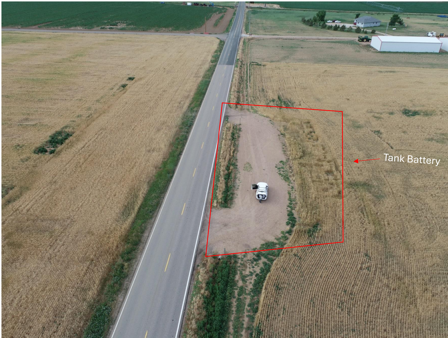
Figure 11: Looking South towards TB, 120 feet in height, Lat/Long: 40.394441/-104.907464.
