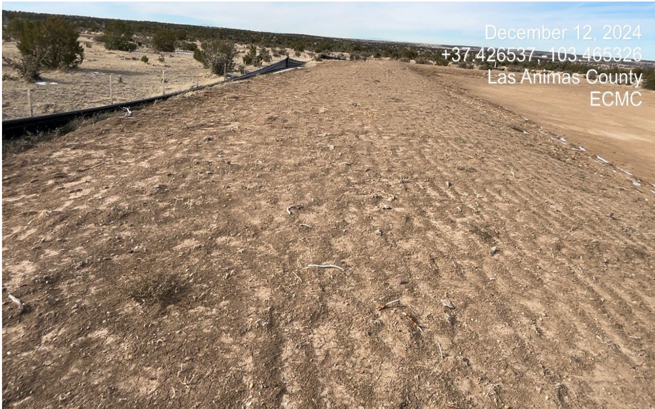
Photo 8. South side of the location facing westtoward the topsoil pile. The topsoil has not been seeded and is not stabilized. The perimeter silyt fence is not maintained.
