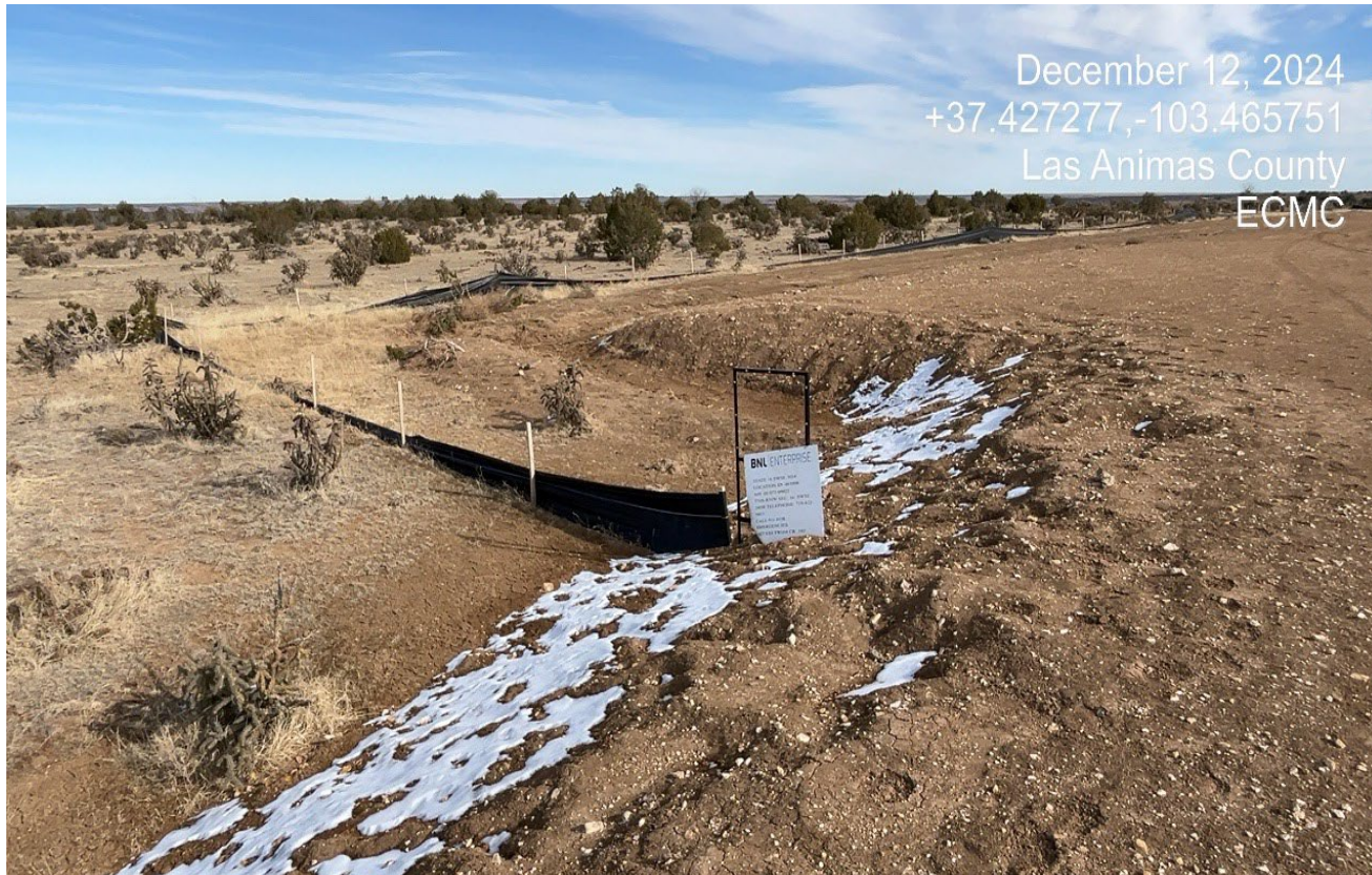
Photo 2. Facing toward the northwest side of the location. The silt fence is not maintained at the location.
