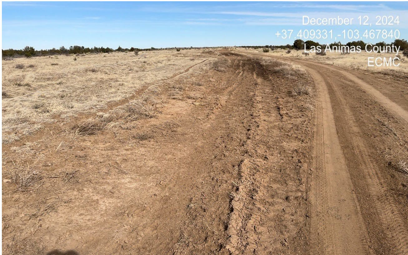
Photo 1. Facing northeast along the access road. There are areas of the road that will need to be repaired and stabilized.
