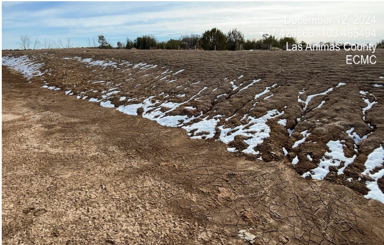
Photo 7. Facing toward the topsoil pile at the south side of the location. There is erosion occurring along the topsoil which is not stabilized or protected..
