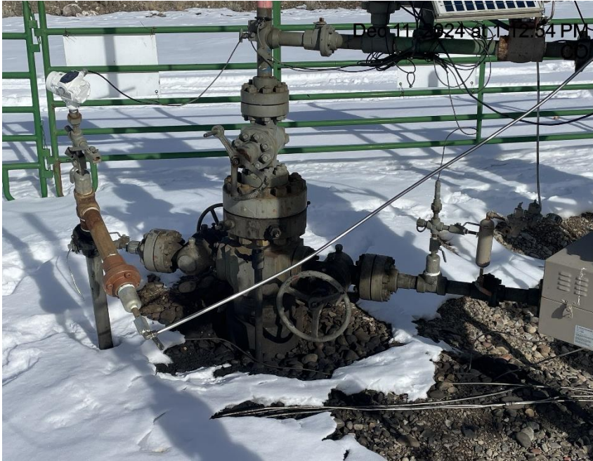
Photo # 3075 Staining around RU 43-6 wellhead
