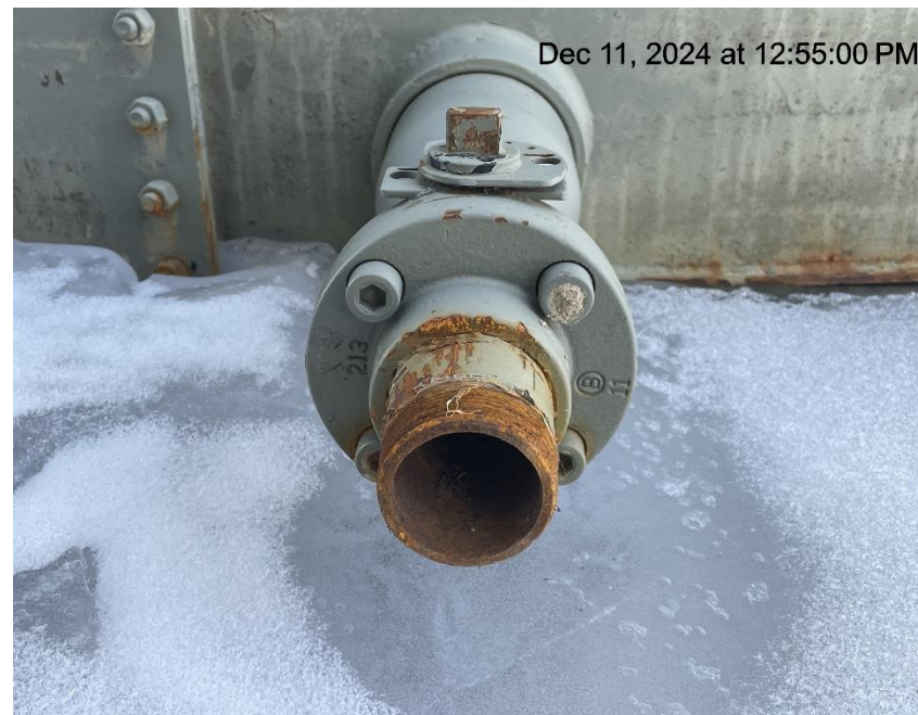
Photo # 3078 Open ended load line
