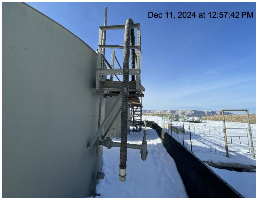
Photo # 3077 Unused hose on tank battery stairs
