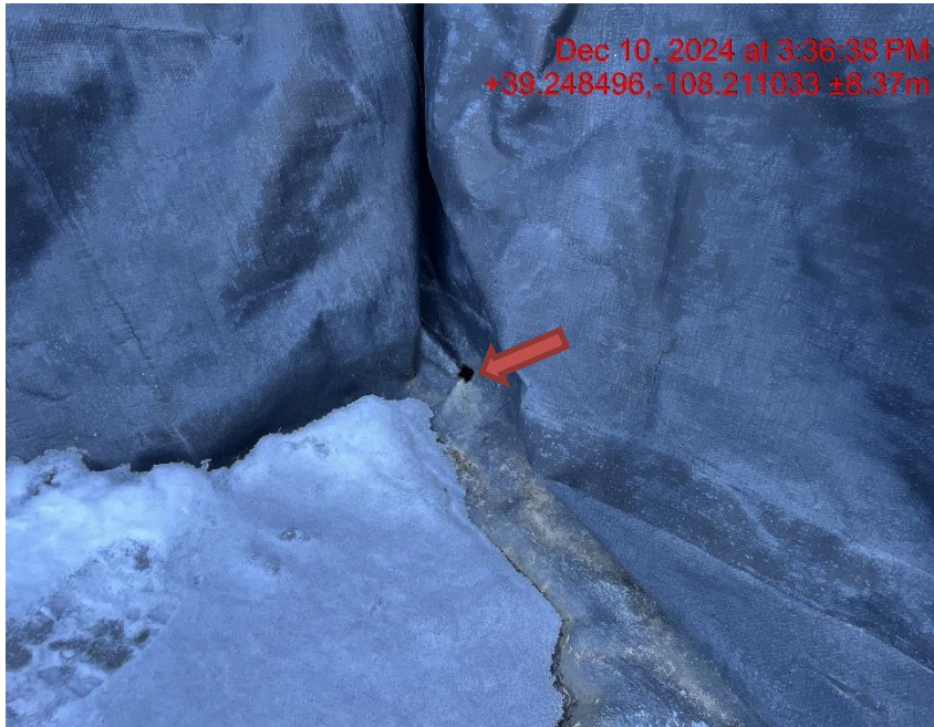
Photo # 0751 Hole in containment liner
