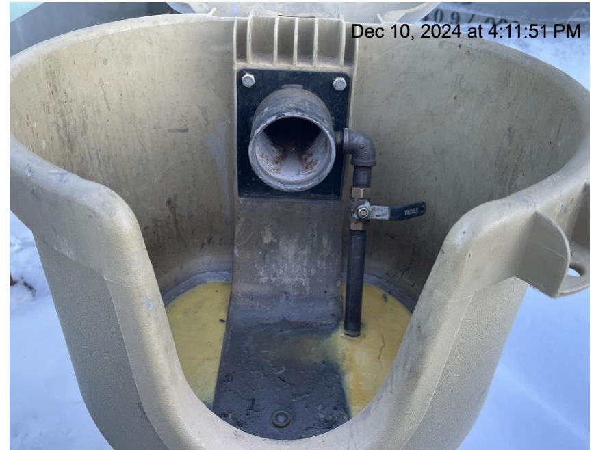
Photo # 2987 Open ended load line
