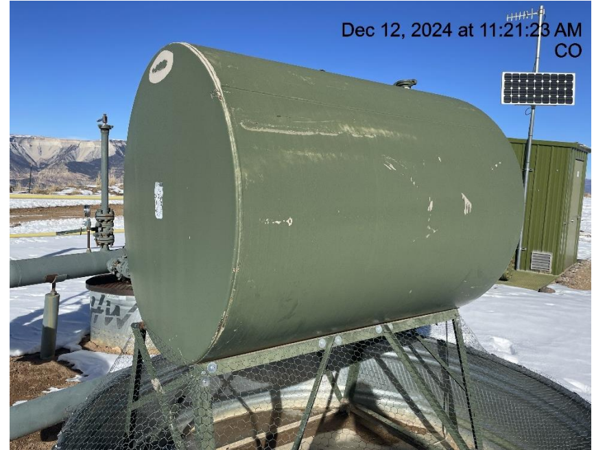
Photo # 3392 Methanol tank improperly labeled/missing some required information
