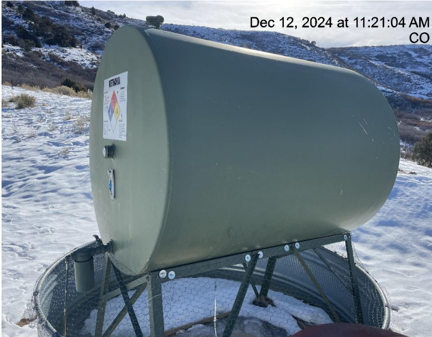
Photo # 3391 Methanol tank improperly labeled/missing some required information
