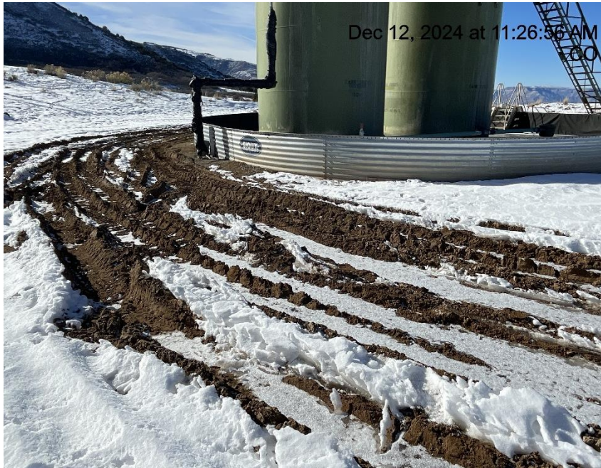
Photo # 3397 Lack of stabilization/compaction
