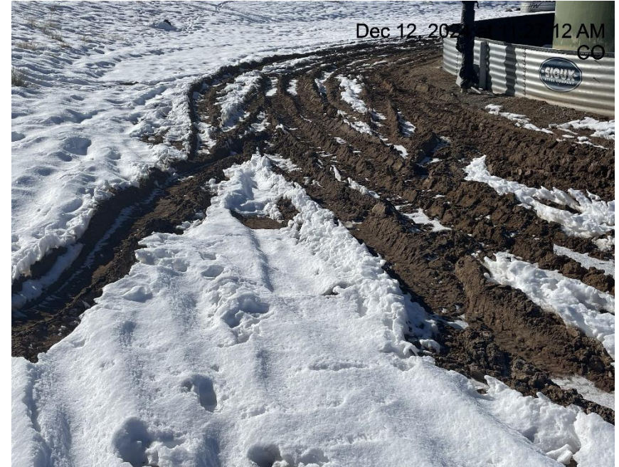
Photo # 3396 Lack of stabilization/compaction
