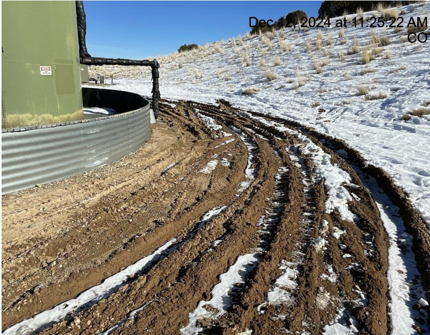
Photo # 3393 Lack of stabilization/compaction
