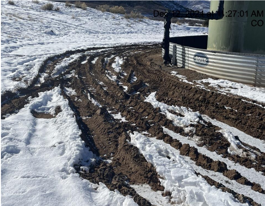
Photo # 3395 Lack of stabilization/compaction
