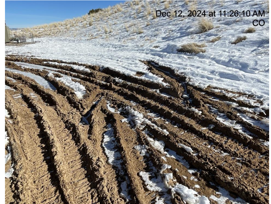
Photo # 3394 Lack of stabilization/compaction
