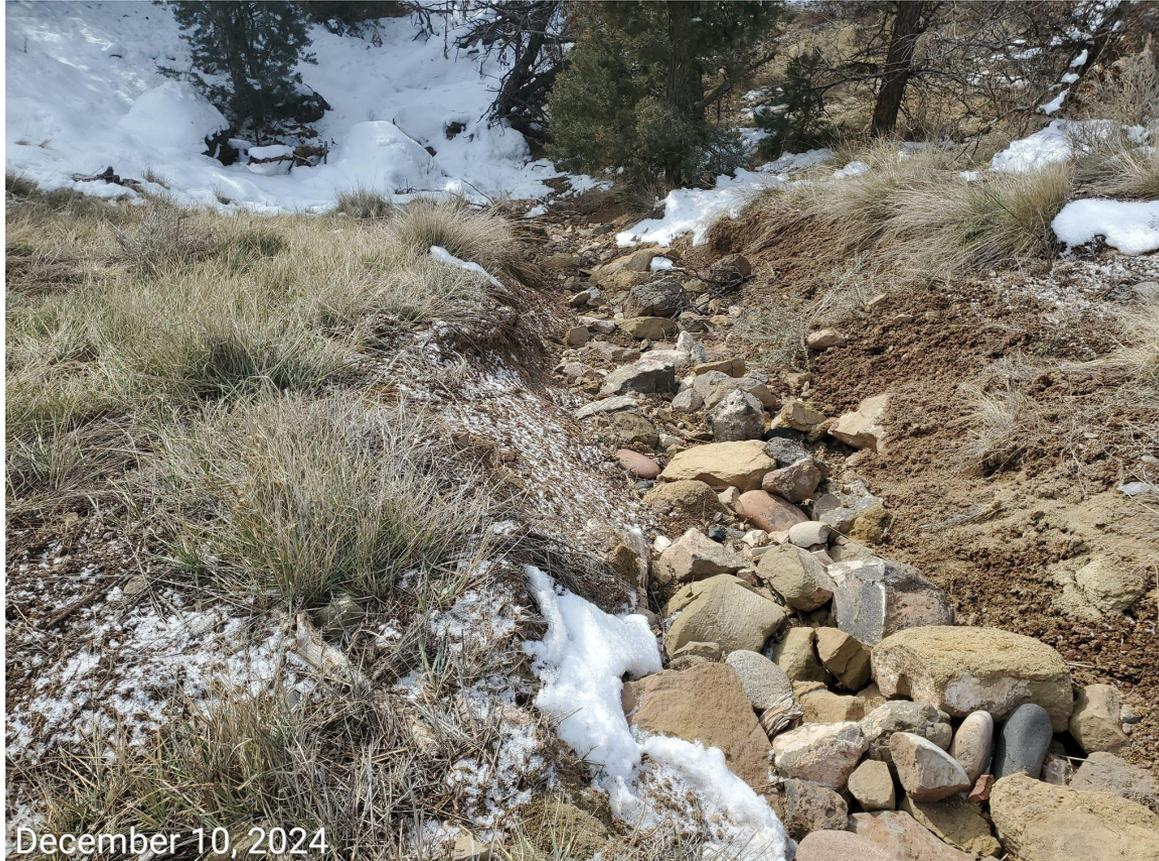
**Photo 6:** Photo taken from below the sediment trap on the southwest end of the Location. Sediment trap has not been installed with a properly engineered outlet; geotextile lining in conjunction with the rip-rap material not observed; slopes within outlet lacks stabilization and erosion degradation / sediment transport is evident
