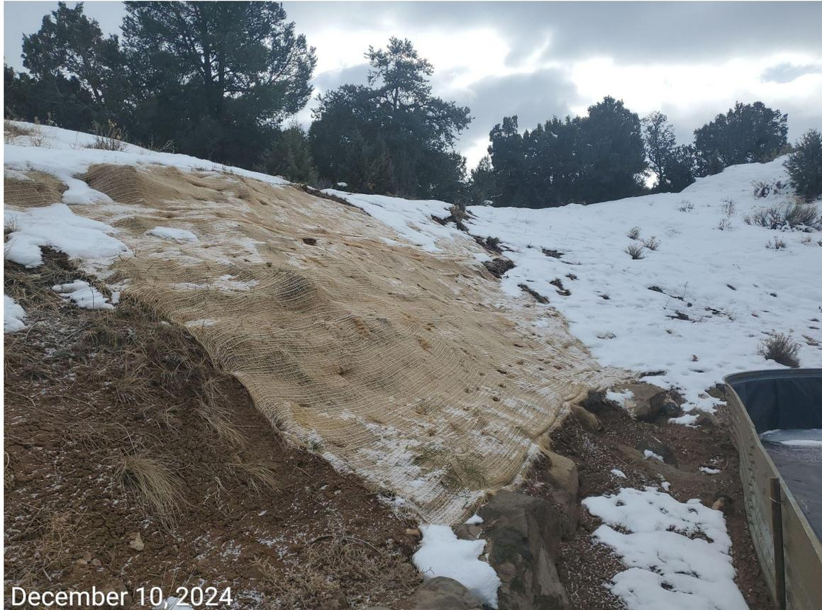
**Photo 2:** Photo taken from east end of the Location. Operator has placed an erosion blanket on a portion of the slopes. BMPs were not evident, or apparent, within remaining areas of concern identified within the previous inspection.
