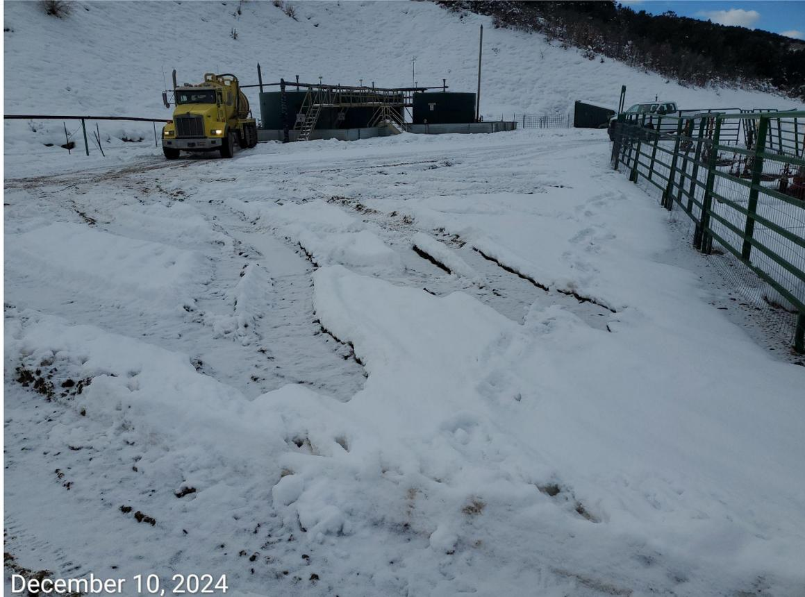
**Photo 3:** Photos 3-5 taken from the working pad surface on the southeast end of the Location. Photos shows tracking/rutting/degradation has persisted on the pad.
